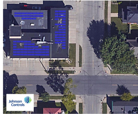
Fire Station #3: 30 kW
