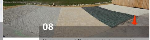
Minimize pavement! When you need it, choose material with openings so water soaks through and doesn't run off.
