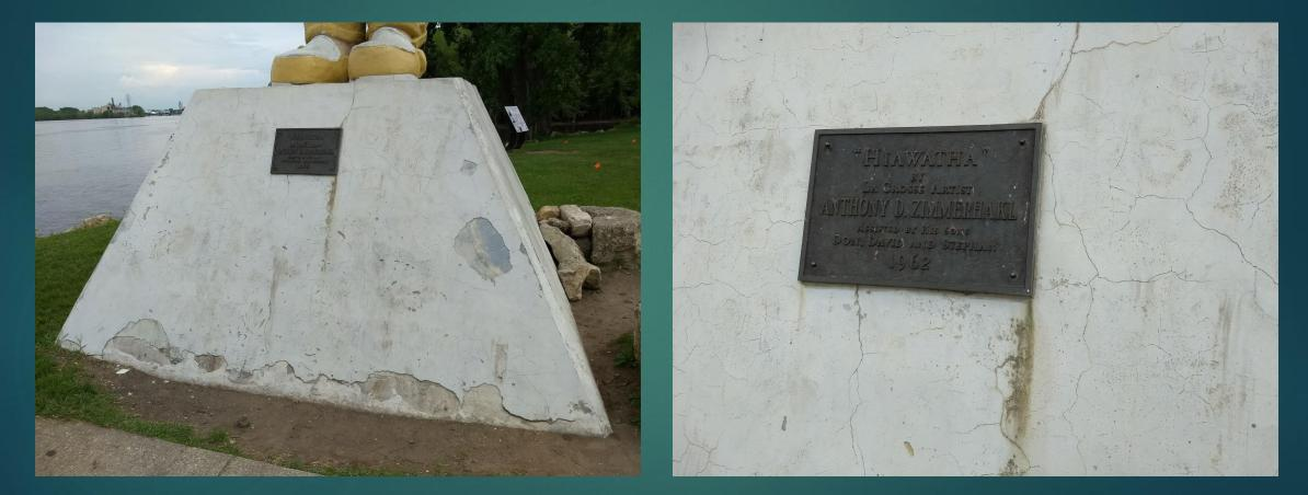
There are numerous spots where the paint has peeled away from the sculpture and significant cracks in the north side as well.
