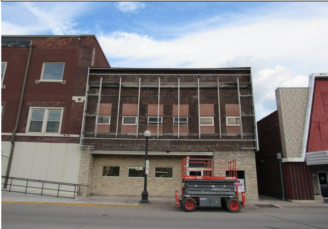
Figure 21 – West Façade during metal slip cover removal. August 2020.
