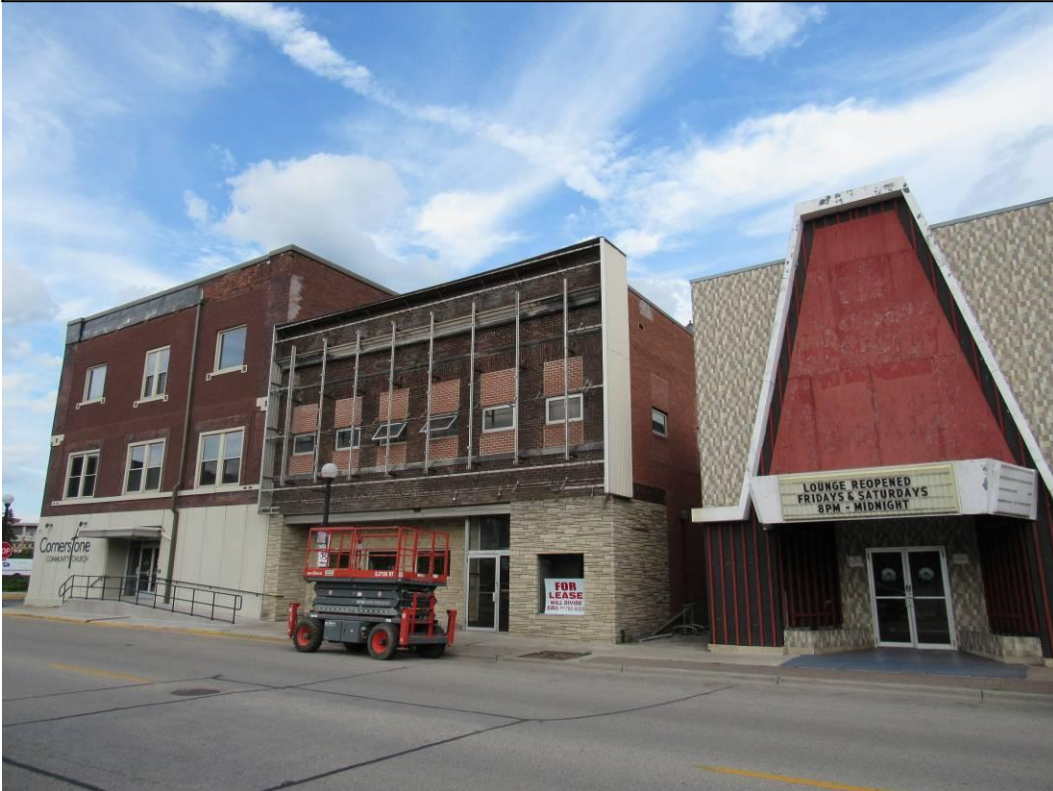
Figure 23 – West Façade during metal slip cover removal. August 2020.
