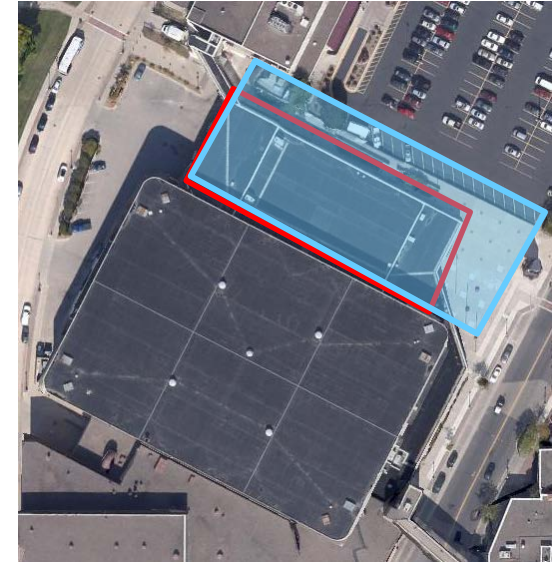
Montgomery Performing Arts Centre (Montgomery, AL) 1,800 seats
