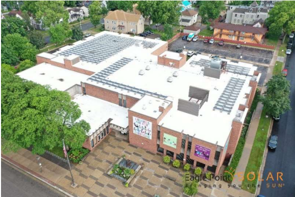
Main Library: 100 kW
