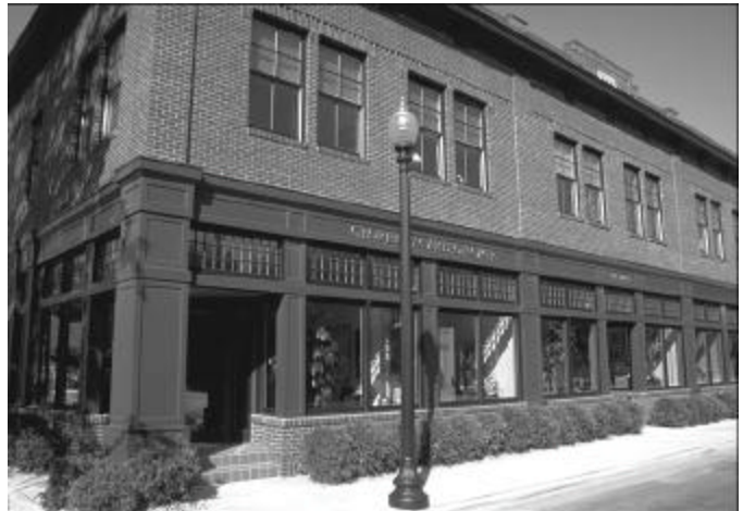
Mixed use building with offices and apartments above storefront shops.
