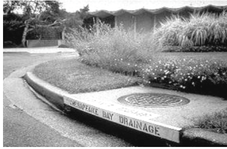
Storm drains can be labeled with stencils to discourage dumping
