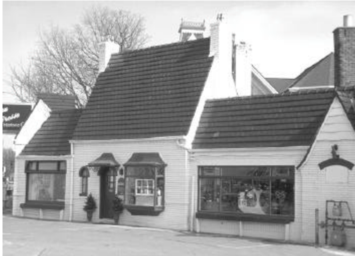
Ott Pure Oil Station – A designated local landmark
