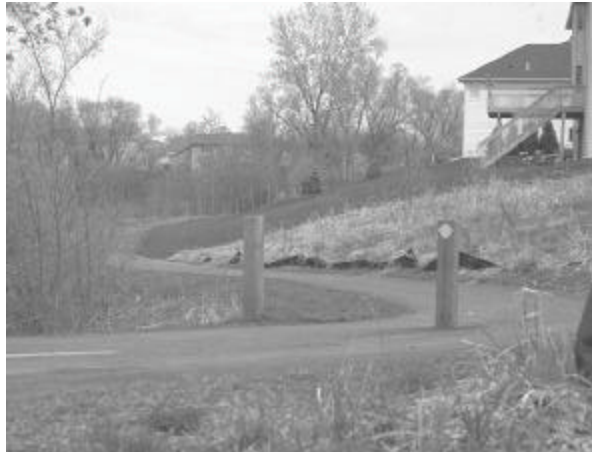
Bike path through new residential development
