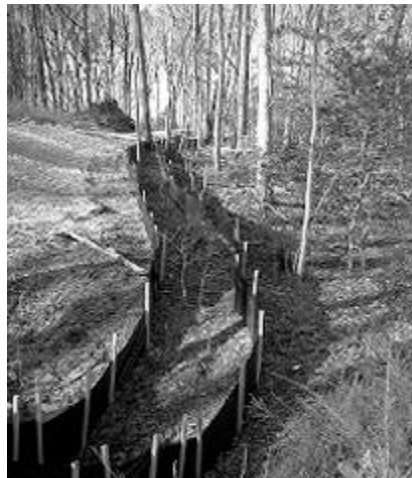
Silt fences prevent the off site transport of sediment
