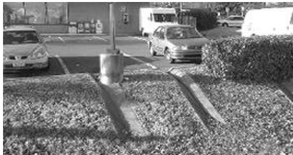
Curb cuts can direct runoff from impervious surfaces to vegetated areas
