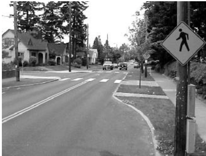
Intersection neck-downs – A traffic calming strategy (i.e.) which reduces pedestrian crossing distance and slows traffic by narrowing site lines, this design is particularly appropriate in high pedestrian areas such as near schools or parks
