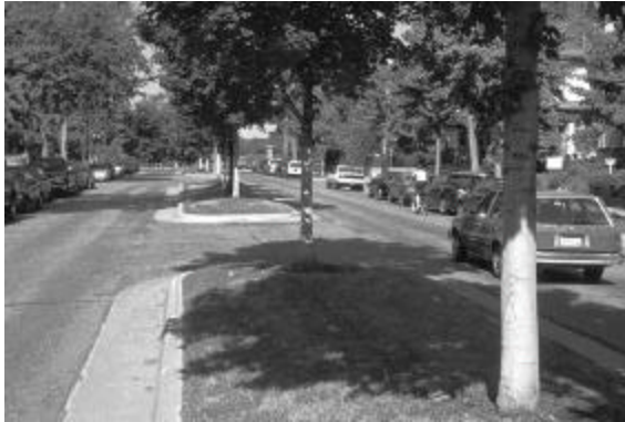
Example of a three lane configuration with one lane in each direction, dedicated left turn lanes, planted medians and parking on both sides
