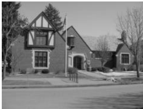
La Crosse Public Library, North Branch, 1941-42, Locally Designated
