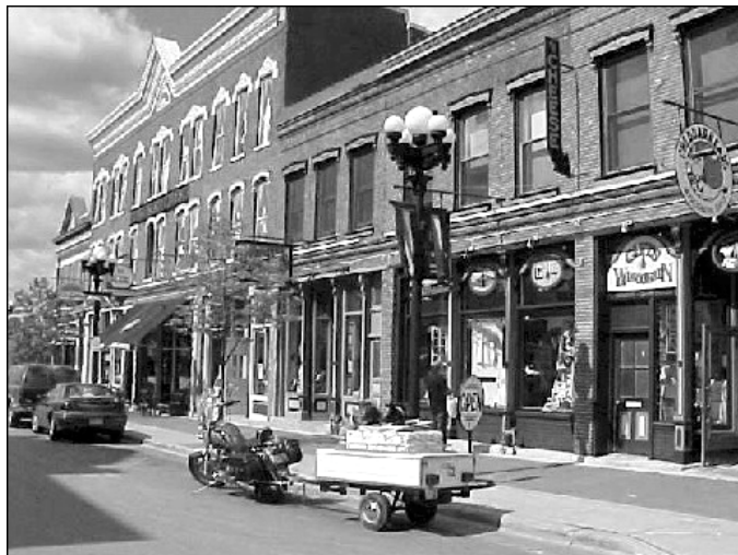
Pearl Street Renovation
