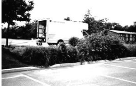
Bioretention areas used in parking areas to collect and treat storm water (Source Univ. of Maryland, 2000)
