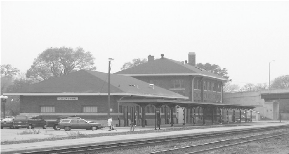
Renovated Amtrak Depot
