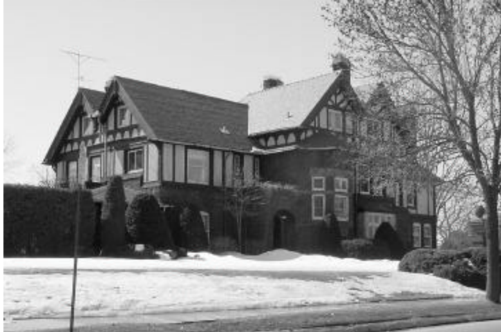
Joseph Hixon House, 1901-02, Cass and King Residential Historic District, NRHP; Locally Designated
