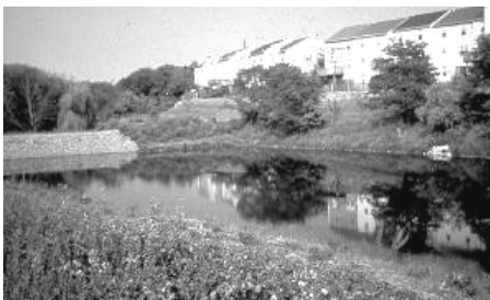
Wet pond detain storm water and facilitate pollutant removal through settling and biological uptake
