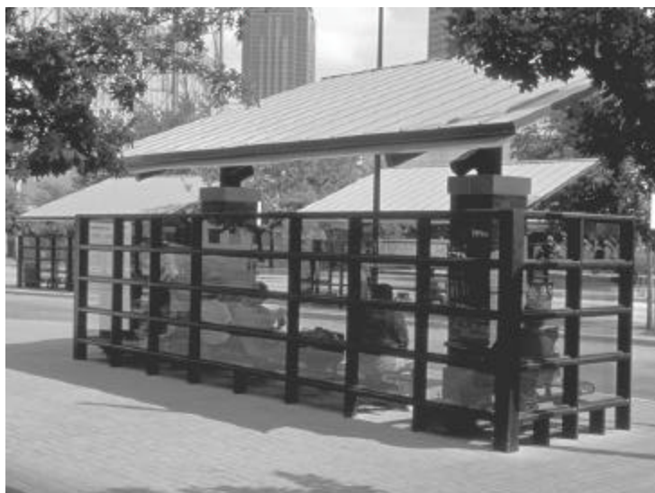
Transit shelters should be attractive and functional
