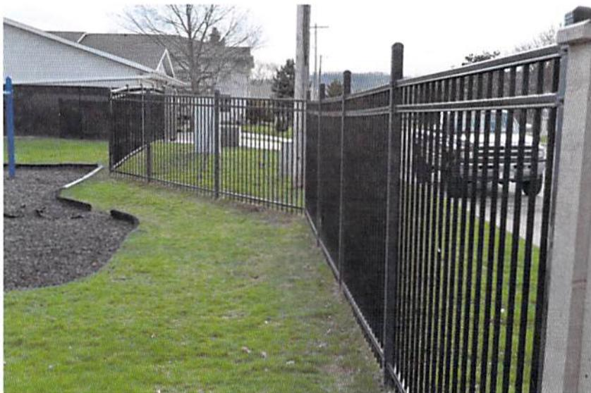
The fire gate, to provide access for fire trucks, is aluminum, as is the adjacent gate for staff to enter/exit in an emergency only.
