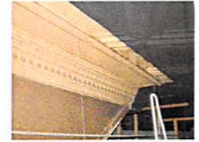
5A PHOTO 1ST FLOOR REUTER-MADER TM CEILING / CORNICE
