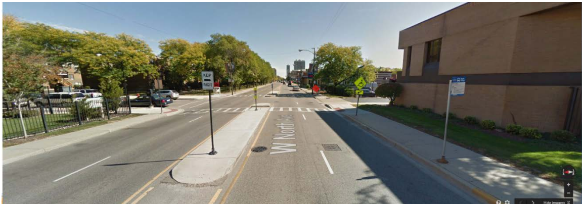
Example of pedestrian refuge islands installed on a four-lane roadway while still permitting left turns. Source: Google.
