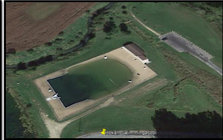
Hokah Swimming Pool- Hokah, MN
