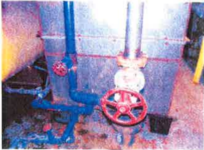
Rusted Pipes Wore Through
