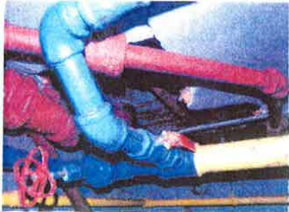
Rusted & Leaking Pipes and Valves
