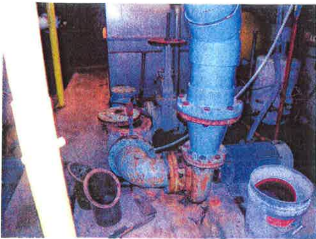
Rusted & Leaking Pipes and Valves
