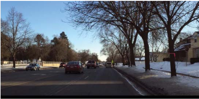
Losey Blvd today
