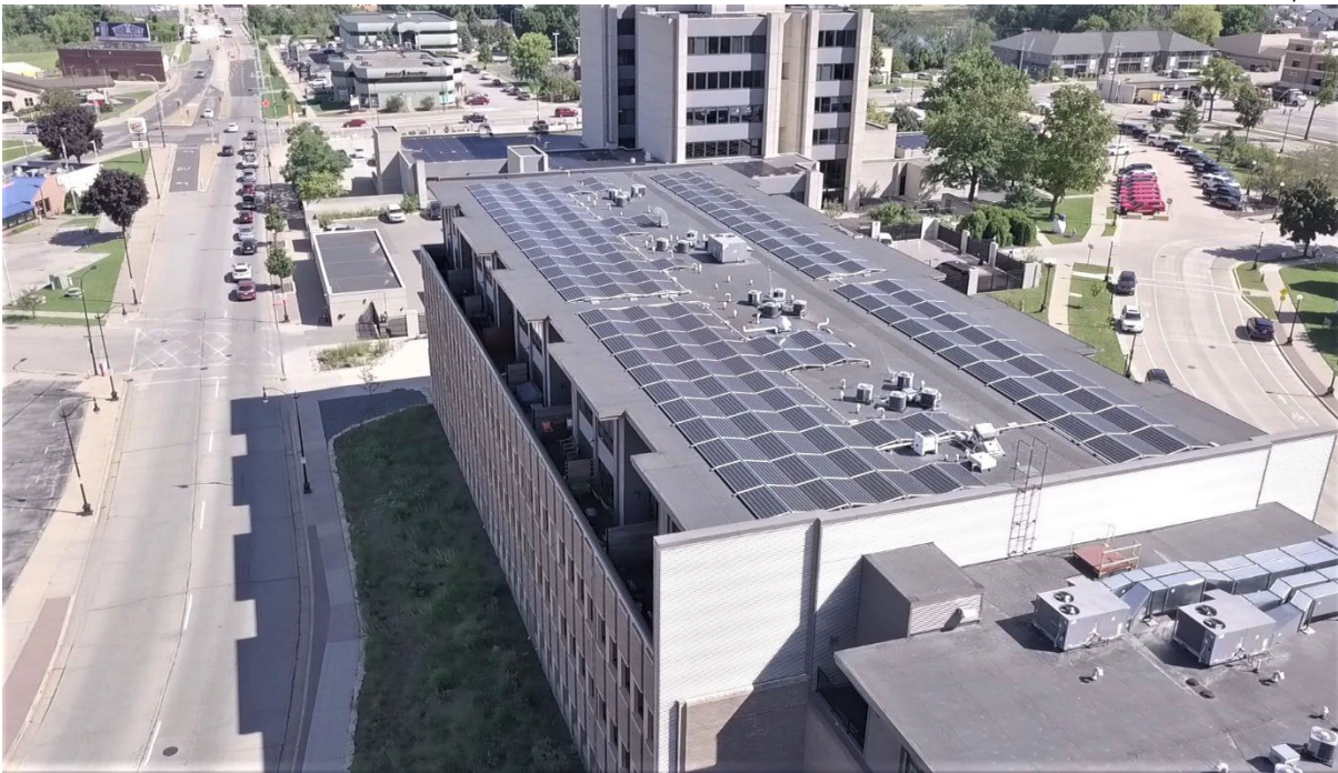
Rooftop Solar Panels – 415 N 6 th St La Crosse, WI The HUB
