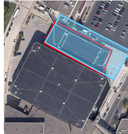
Montgomery Performing Arts Centre (Montgomery, AL) 1,800 seats
