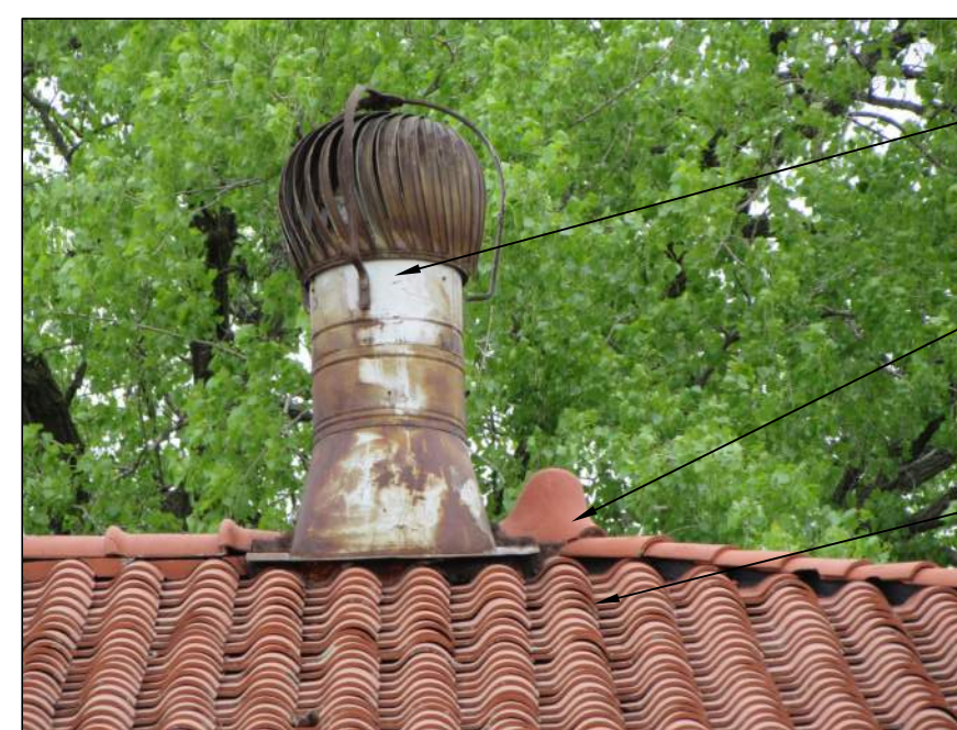
P2 ROOF VENTILATOR NO SCALE
