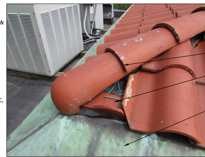
P7 TYP. HIP TILE NO SCALE
