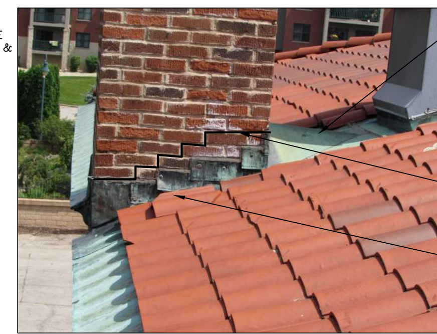
P11 FLASHING @ CHIMNEY NO SCALE
