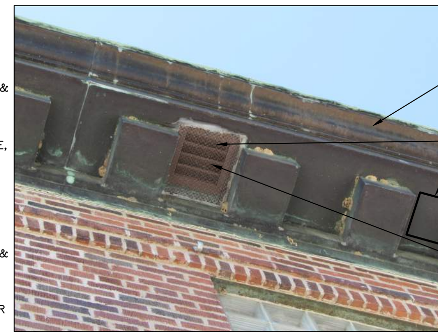
P5 TYP. SOFFIT VENT NO SCALE
