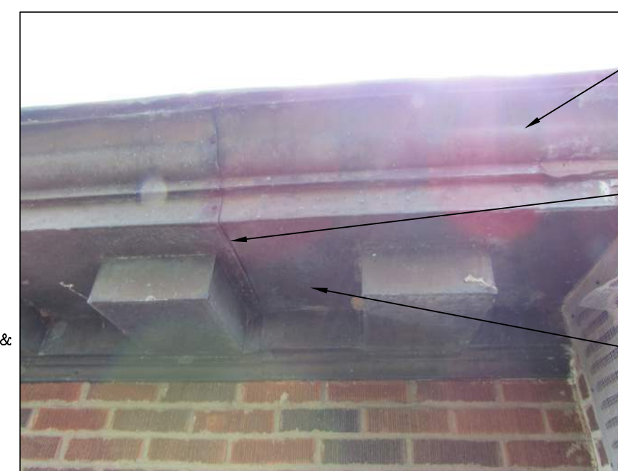
P6 CORNICE SEAM NO SCALE
