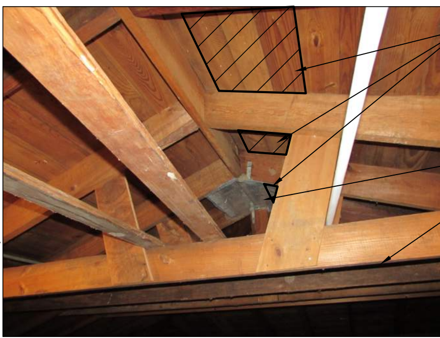
P12 TYP. RIDGE FRAMING NO SCALE
