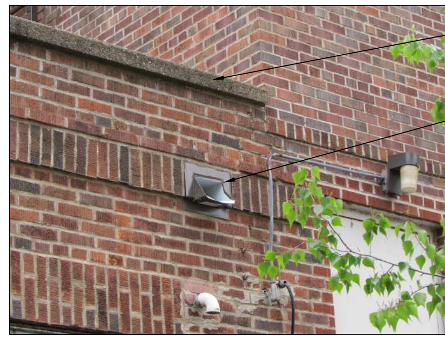
P3 TYP. SCUPPER NO SCALE
