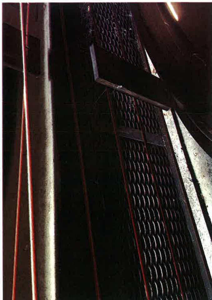
Roof access through grate on Level 2
