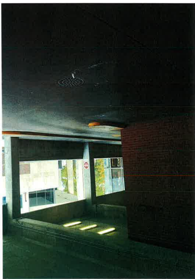
Ceiling drains near floor drain
