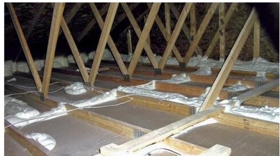
When insulating an attic, always aim to seal the various gaps and air passages that allow conditioned air to leave the home. Around wires, pipes, chimney chases, the hatch/entrance and drywall top plates. Sealing after insulating is hard.
