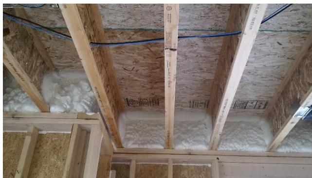
In years past, people often put fiberglass batts into rim joists. The issue is that fiberglass rarely is put in for a perfect fit, and is also not air-tight. Because of which, outdoor air can leak in (And pests can sometimes enter too). Replace fiberglass with rigid or spray foam insulation, and once that air tight barrier is put in you can add fiberglass if desired.
