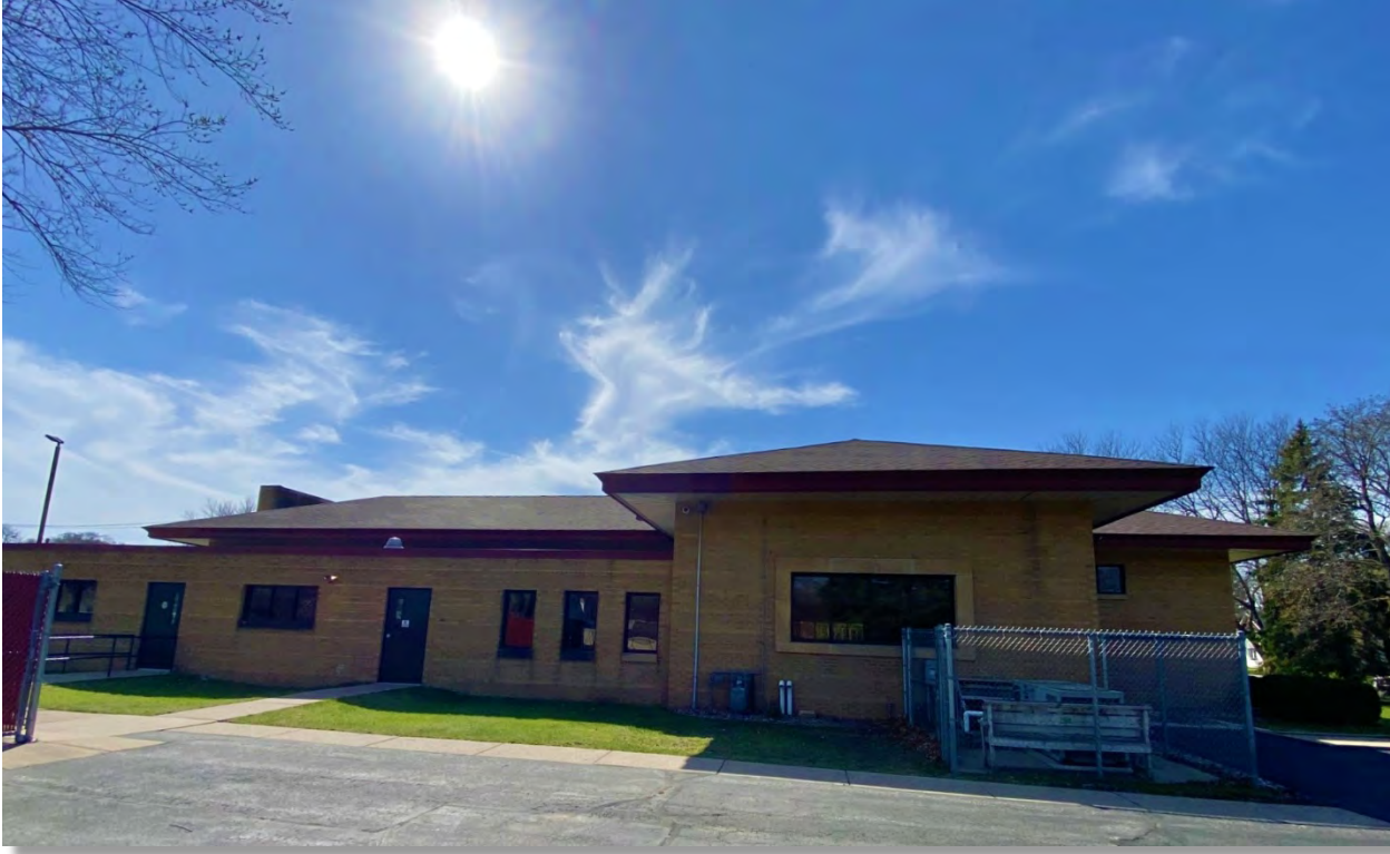
South Branch Library, East Elevation, 2024. Source: David Riel.
