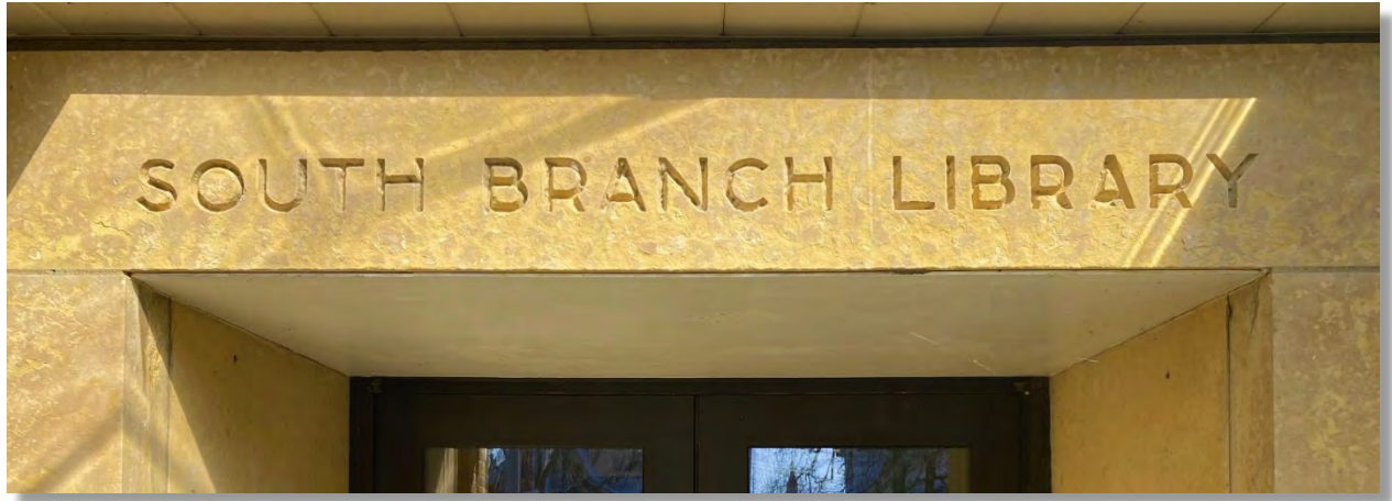
South Branch Library, Carving Detail, 2024. Source: David Riel.
