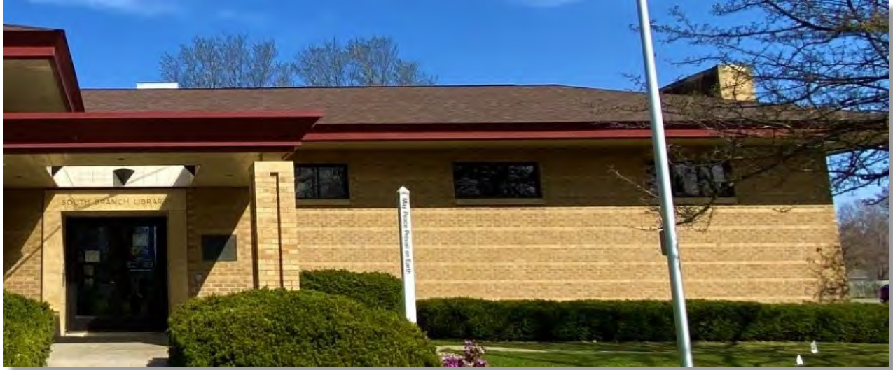
South Branch Library, Window Detail, 2024. Source: David Riel.
