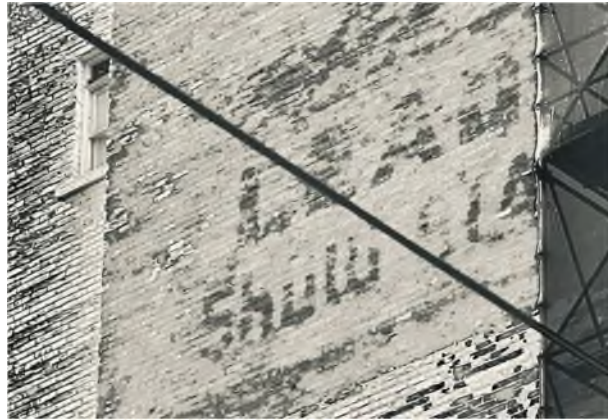
Photograph of the Queen Street "Loew's" sign before the Restoration Project
