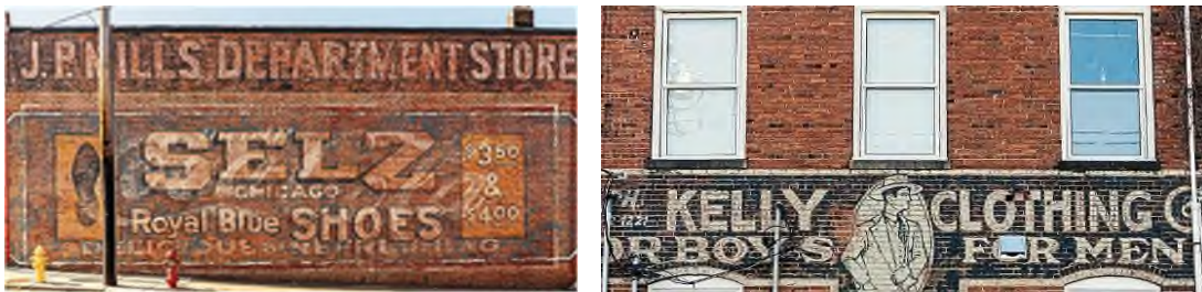
“Selz Chicago” and “Kelly Clothing” signs after the 2020 restoration project
