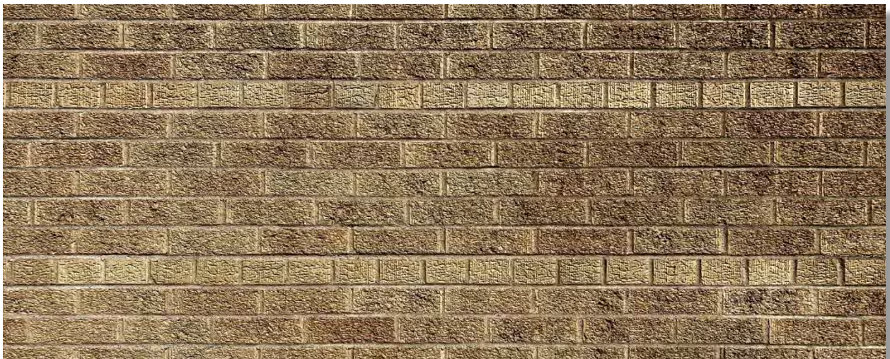
South Branch Library, Brick Detail, 2024. Source: David Riel.
