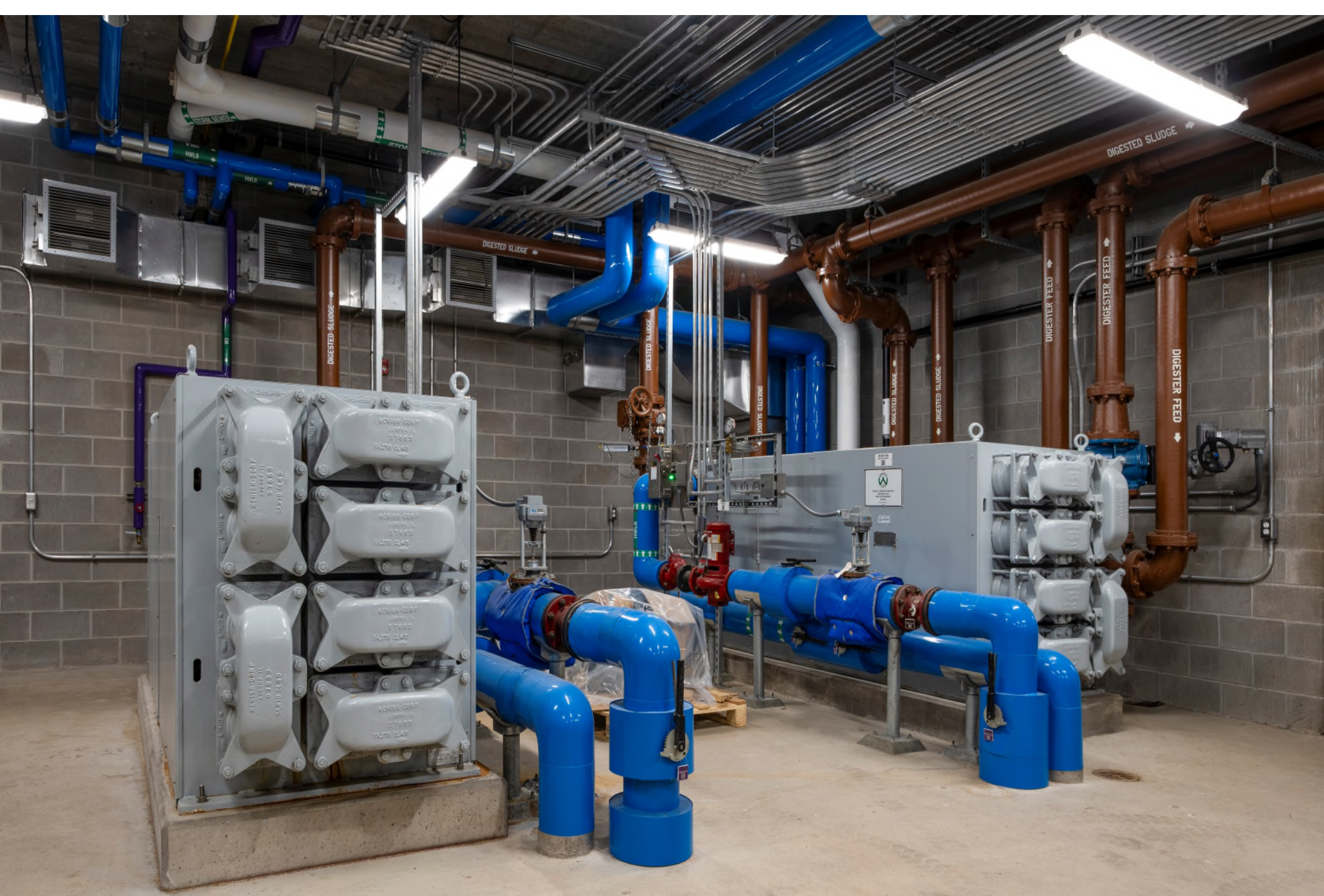
Dedicated heat exchangers for each anaerobic digester
