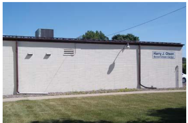
Exterior lighting fixtures. (2012)
