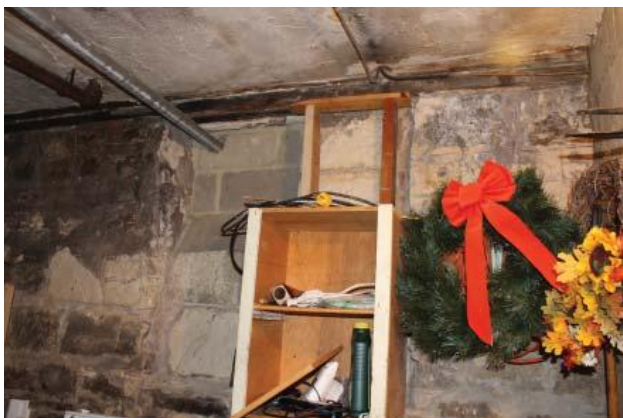
Foundation condition in lower level storage area. (2012)
