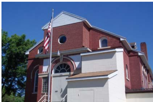
Exterior lighting fixtures. (2012)
