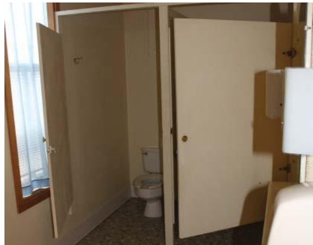
Partition obscuring restroom window. (2012)
