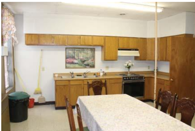
Second floor kitchen with vertical tie rod. (2012)
