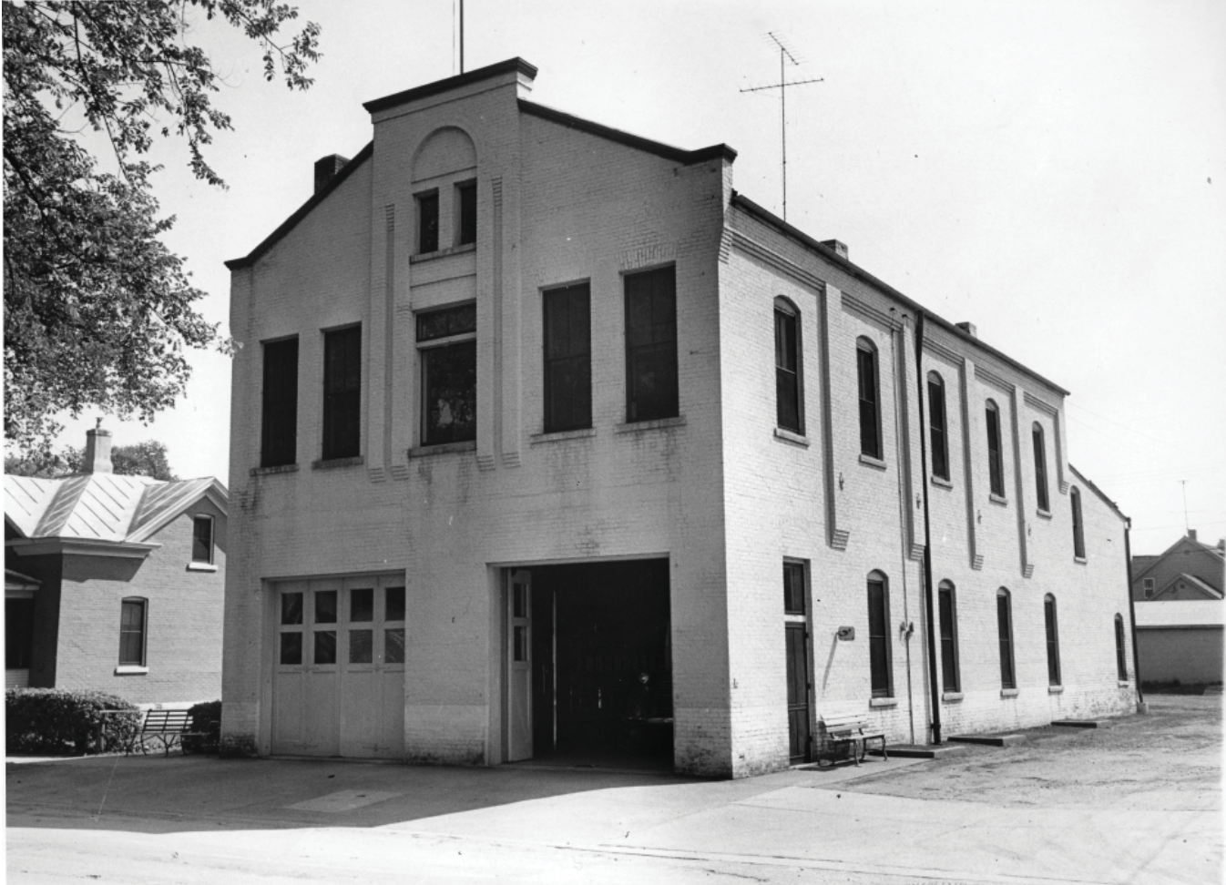
Fire Station #5 (c.1960)
