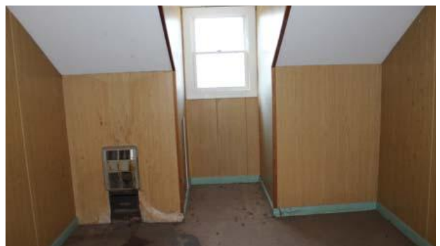
Finished storage space on second floor. (2012)
