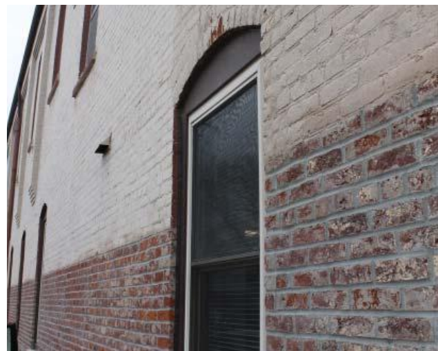
Cleaned and re-tuckpointed brick. (2012)
