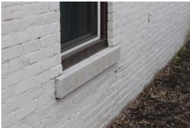
New stone sill in painted brick wall. (2012)
