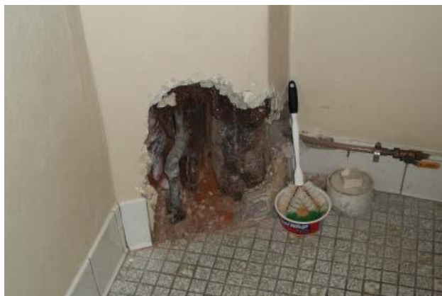
Opening in wall to access piping. (2012)
