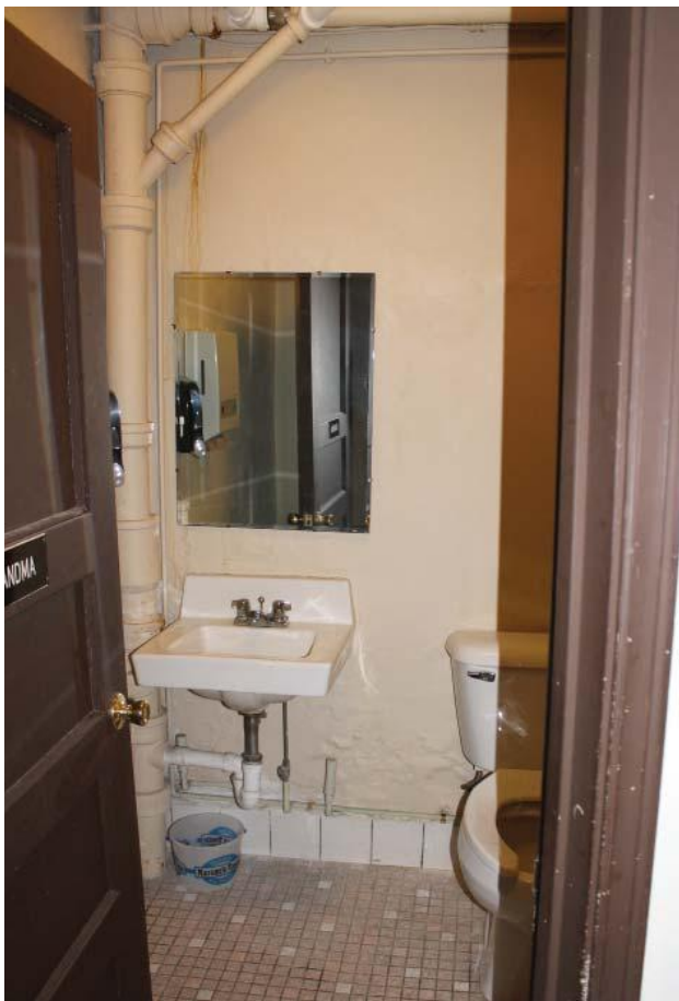
Lower level rest rooms in lower level. (2012)
