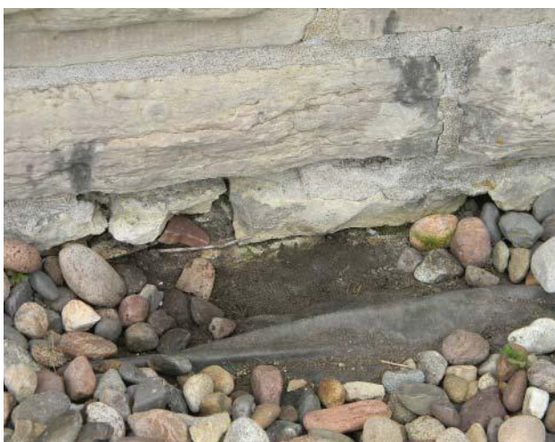
Close-up of limestone wall foundation at grade on the west elevation.
