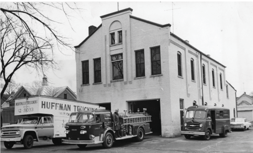
Fire Station #5 (c.1960)
