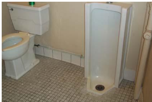
Lower level men's room in original building. (2012)
