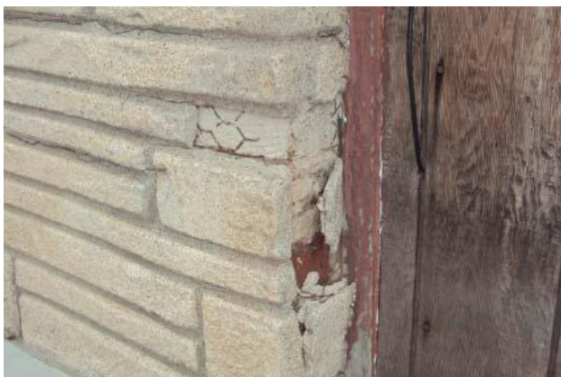
"Stone" patterned stucco on main facade. (2012)
