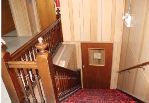
Added enclosure to central stair from second floor. (2012)
