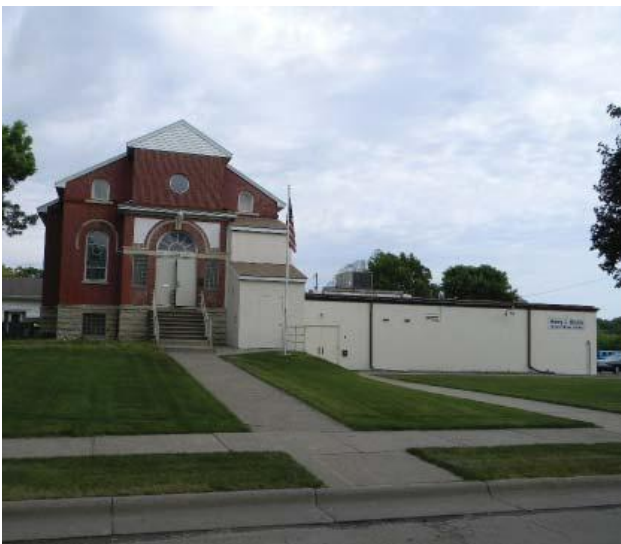
South Elevation showing original building and 1975-80 additions.
