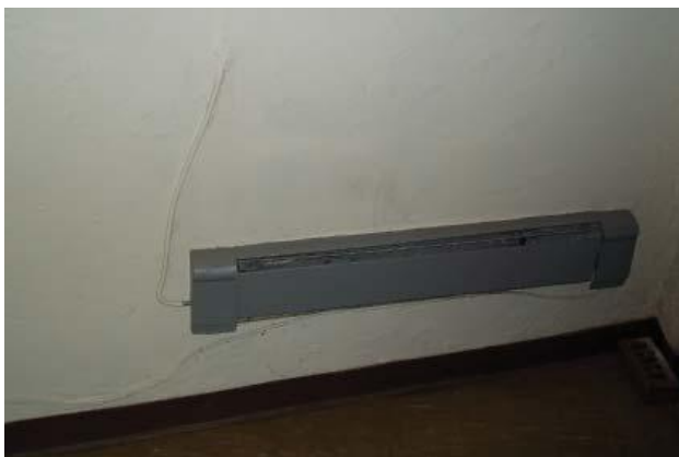
Supplemental electric heat. (2012)
