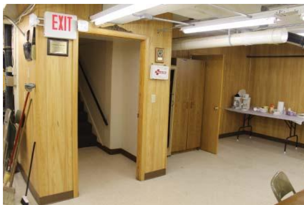
Central egress stair from basement. (2012)
