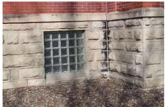
Foundation and Sill condition at south elevation (2012)
