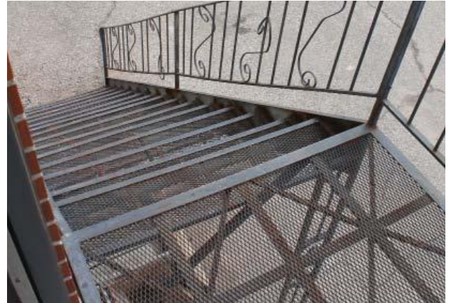
Fire escape stair at south end of building. (2012)
