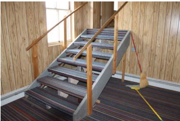
Stair from south meeting room to second floor hall. (2012)
