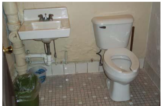
Lower level women's room in original building. (2012)
