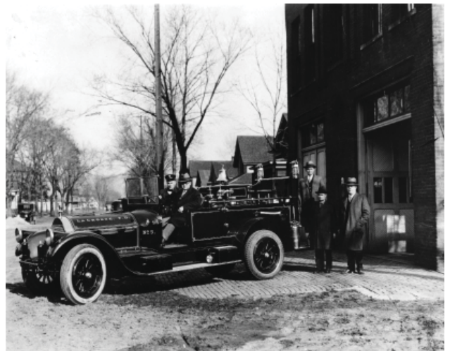
North elevation with new fire truck and Mayor Verchota (4/18/1926)
