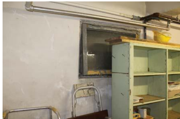
South west storage room, exterior window. (2012)
