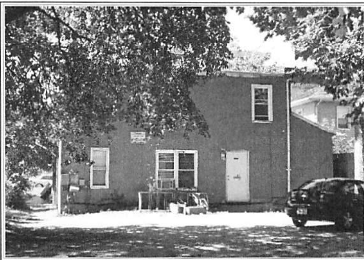
Subject Exterior Rear Exposure Camera Facing Westerly
