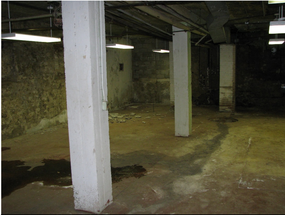
Figure 16 – Concrete columns and slab in basement. January 2017.
