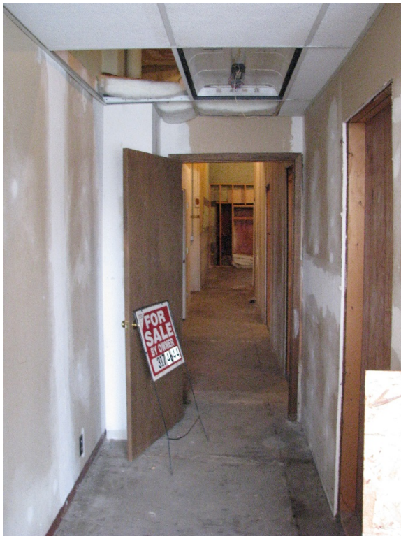
Figure 21 – First floor looking south. January 2017.
