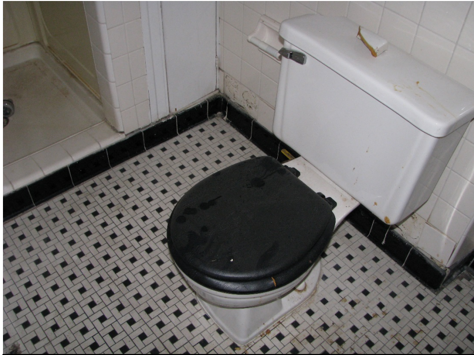
Figure 27 – Typical second floor restroom. January 2017.
