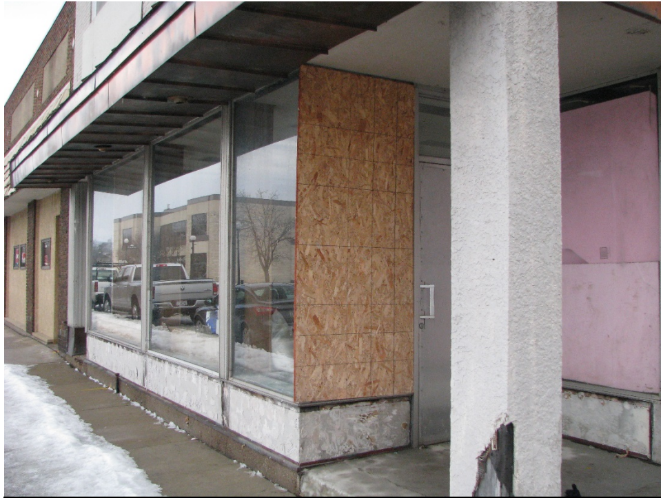
Figure 13 – Detail of modern storefront. January 2017.
