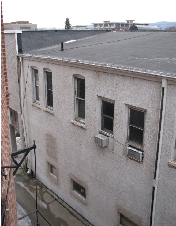
Figure 14 – West façade of 514 State Street. January 2017.
