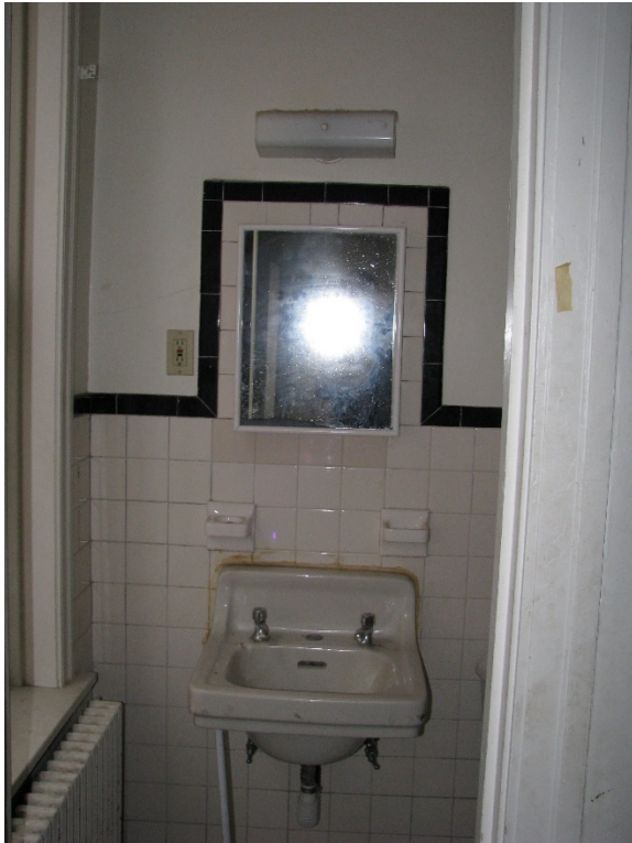
Figure 23 – Typical second floor restroom. January 2017.
