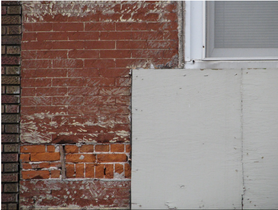
Figure 31 – Test patch of brick restoration treatment. September 2017.
