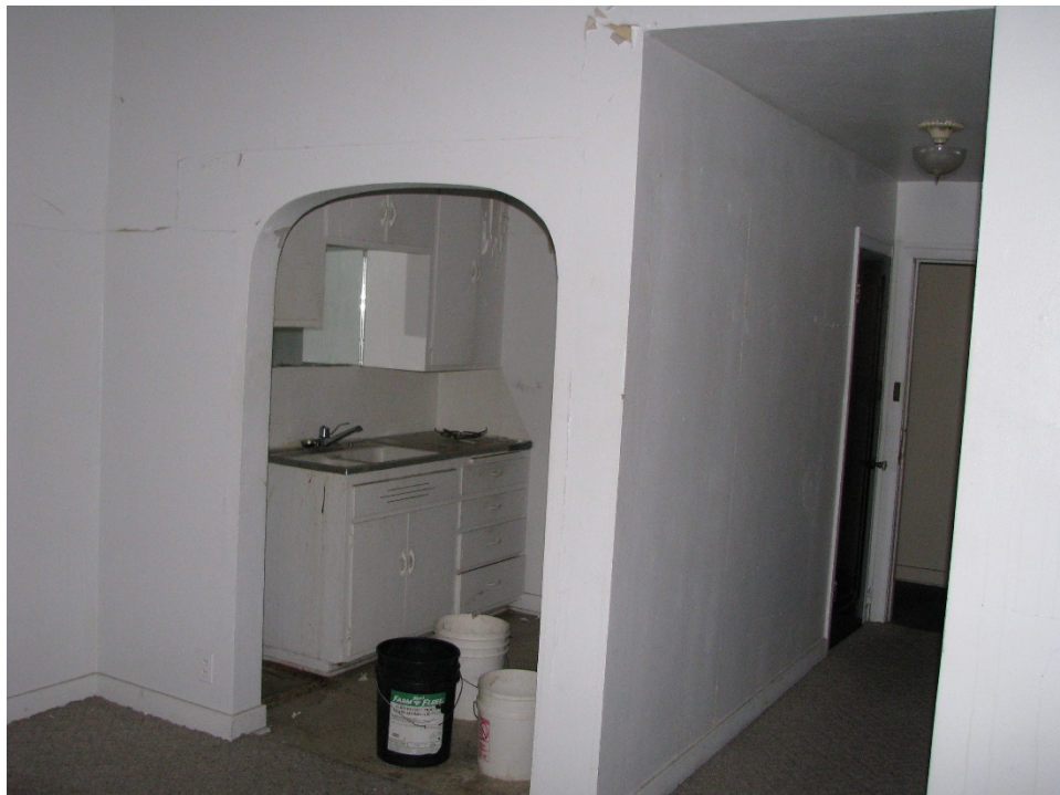
Figure 28 – Typical second floor kitchen & entry hall. January 2017.
