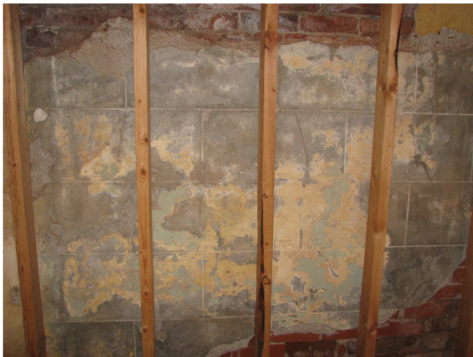
Figure 19 – Decorative scored plaster work on first floor. January 2017.
