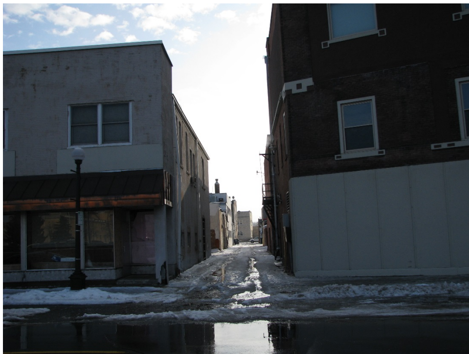
Figure 10 – Alley west of 514 State Street. January 2017.
