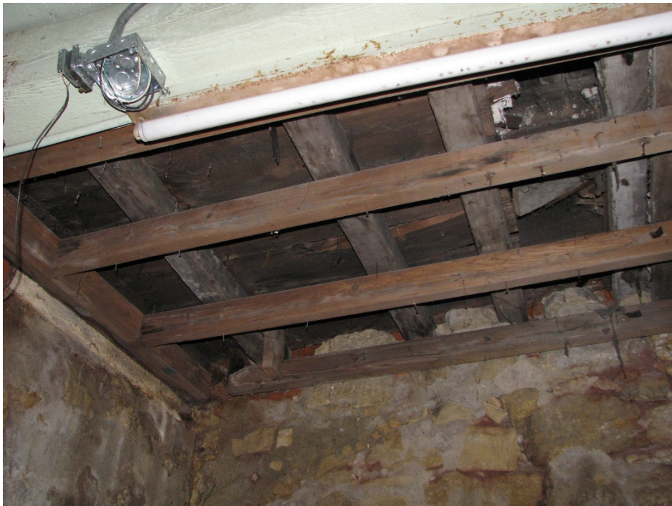
Figure 17 – Wood floor framing below stair to second floor. January 2017.
