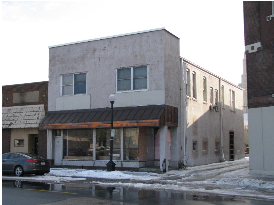
Figure 9 – North (Front) façade of 514 State Street. January 2017.
