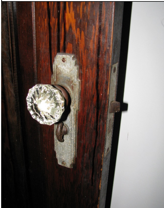
Figure 25 – Apartment entry door hardware. January 2017.
