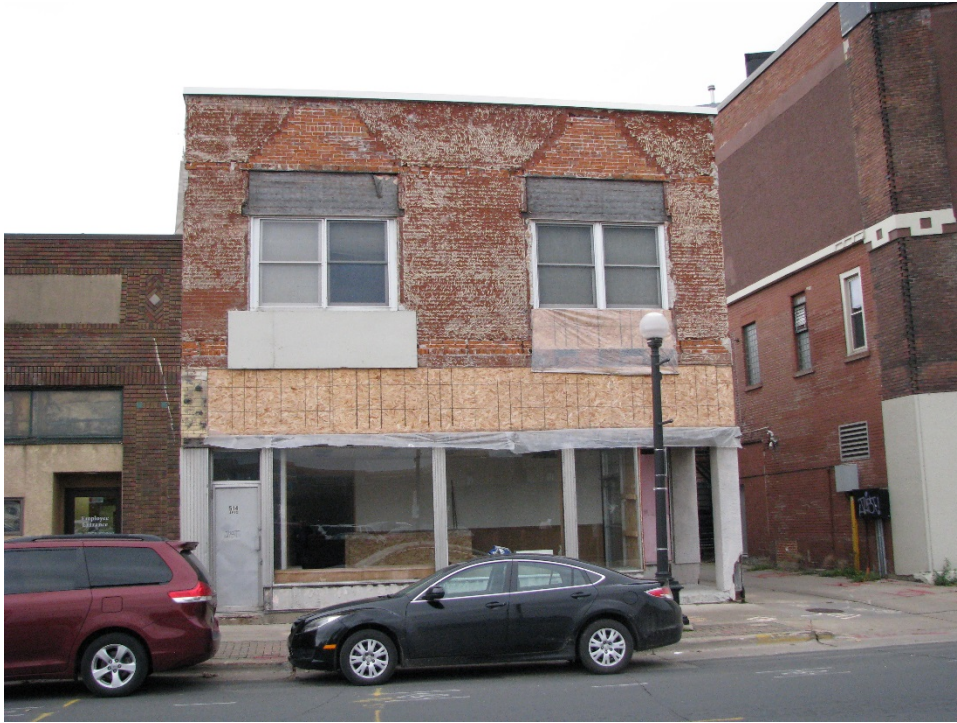
Figure 29 – North (Front) façade after stucco removal. September 2017.
