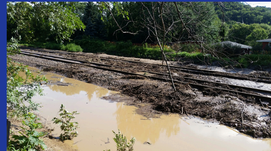
Stormwater utility monitoring flooding at Ebner Coulee Drainage Ditch, 2017
