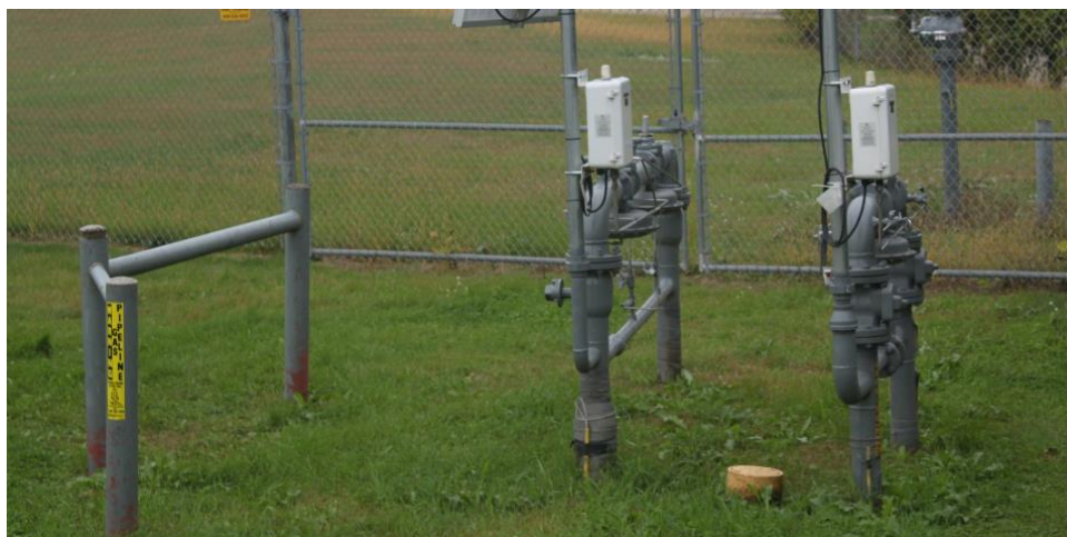
Xcel Portion of the Site
