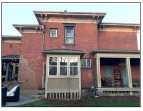
The applicant has stated that the existing footings are structurally inadequate to support the porch and need to be replaced. The main porch supports are deteriorating and are also structurally inadequate and need to be replaced. The existing windows and doors would be replaced and the exterior walls would be rebuilt and sided with fiber cement board siding. The existing steps and porch roof would remain.
