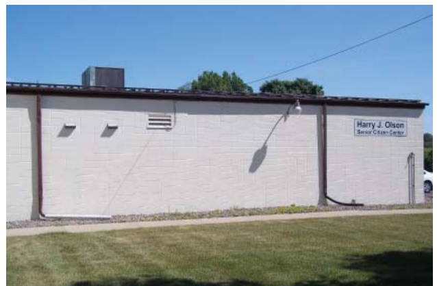
Exterior lighting fixtures. (2012)
