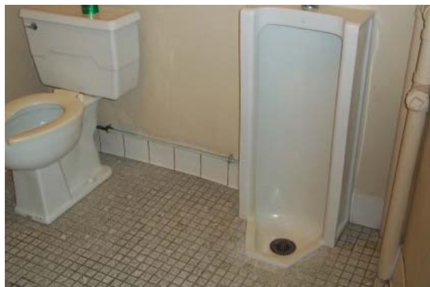
Lower level men's room in original building. (2012)
