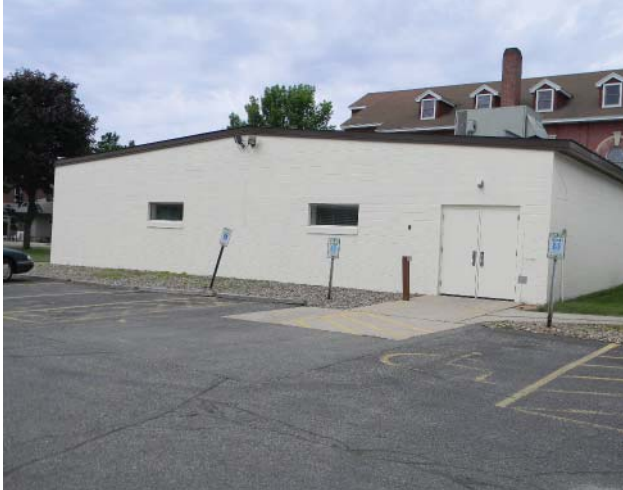
East wall of 1975 addition with original building behind.
