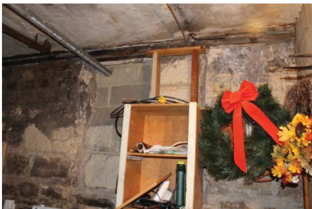
Foundation condition in lower level storage area. (2012)
