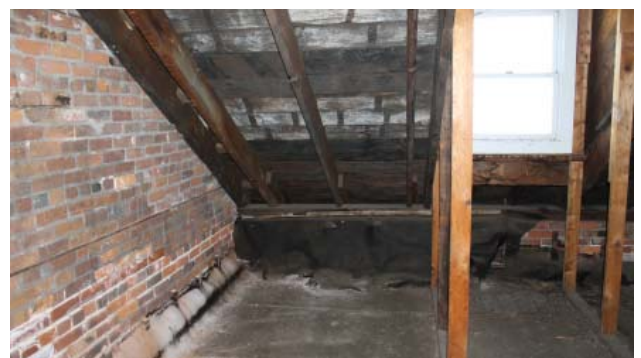
Un-finished space on second floor. (2012)
