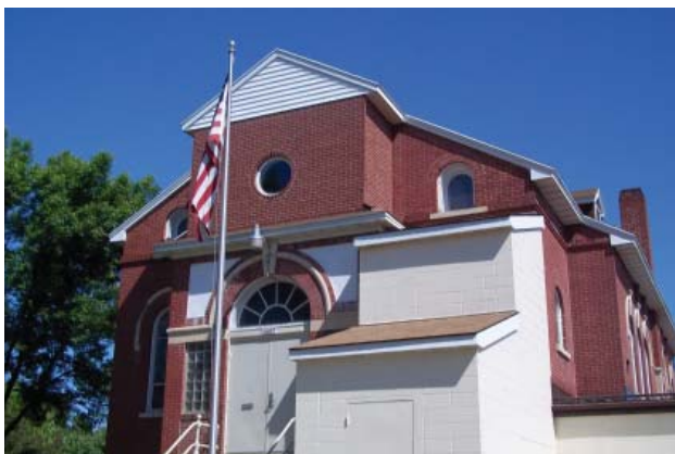
Exterior lighting fixtures. (2012)
