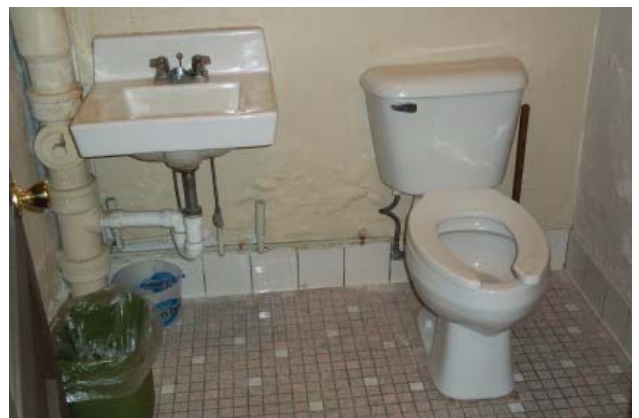
Lower level women's room in original building. (2012)
