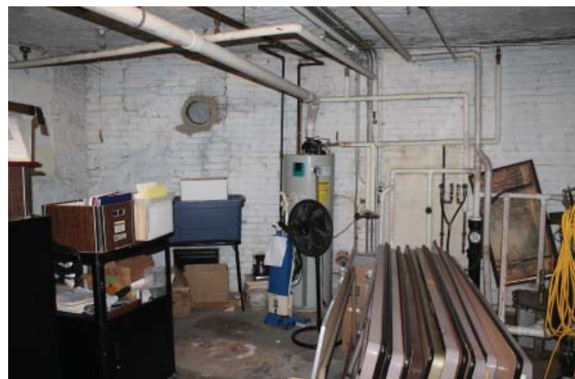
Interior wall condition in lower level storage area. (2012)
