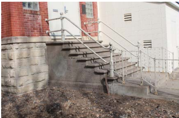
Brick and Foundation condition at south elevation (2012)
