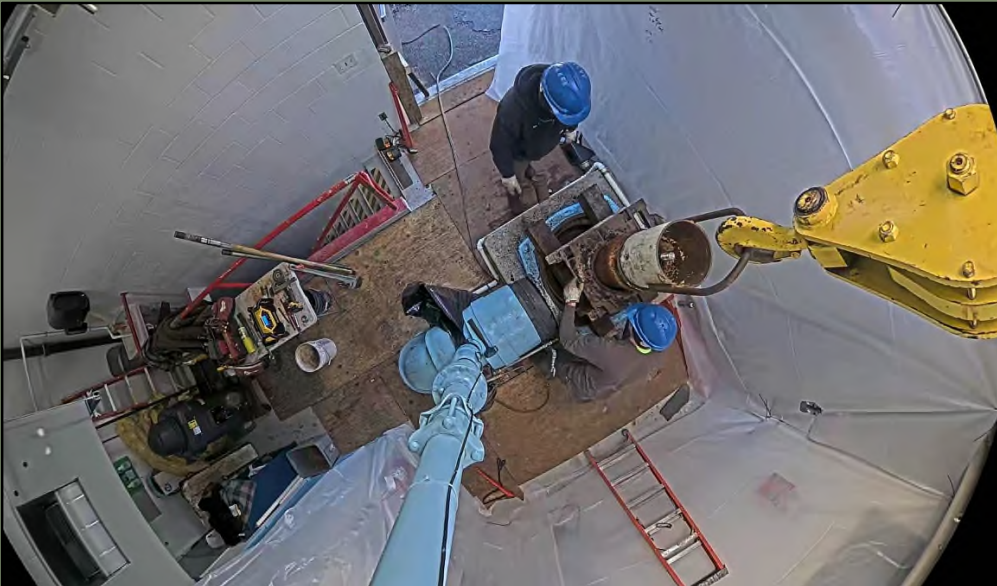
Well 16 Pump Being Pulled in 2025
