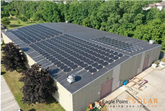
Municipal Service Center: 100 kW
