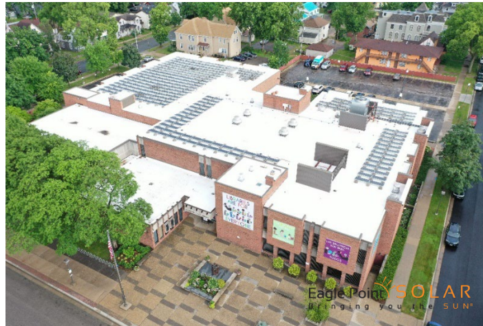
Main Library: 100 kW
