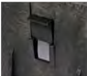
Temporary drop port
