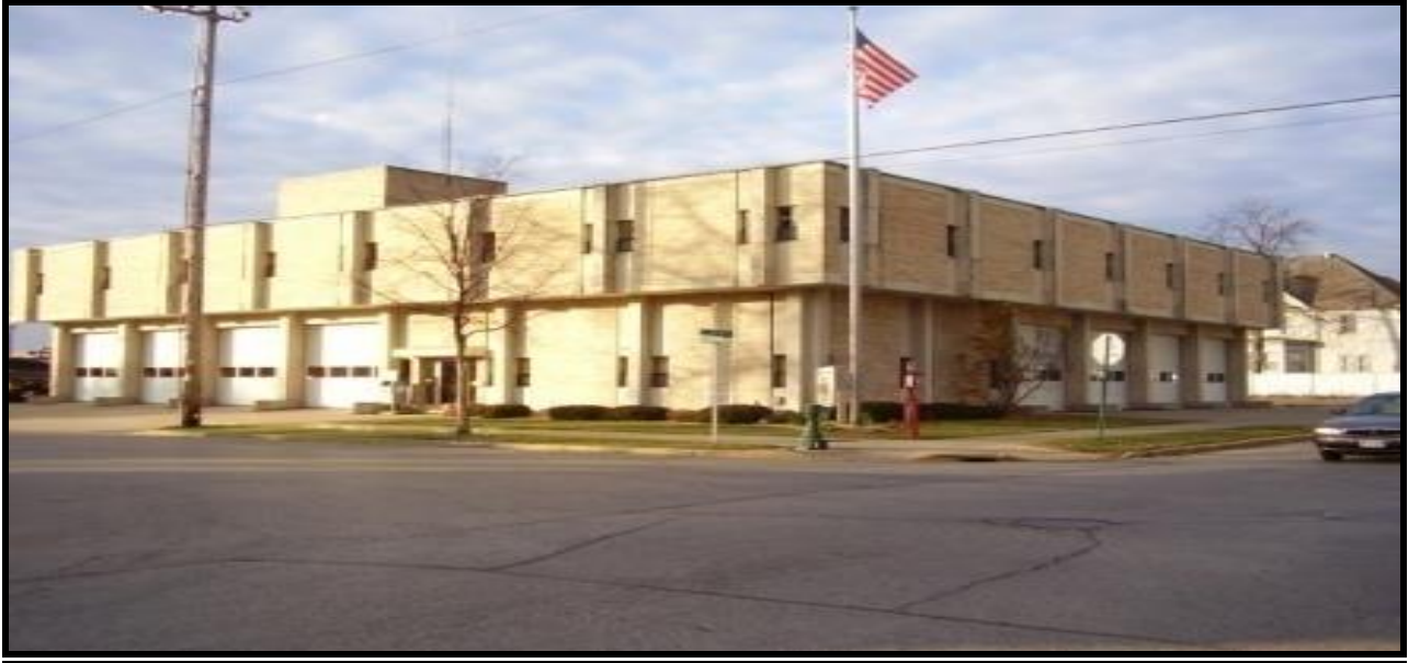
Station 1 at 726 5 th Avenue South – built in 1967 (Downtown District)
