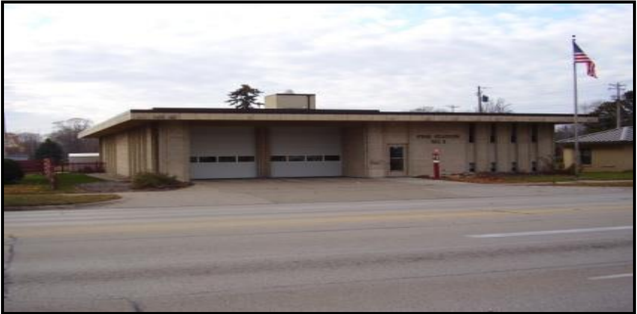
Station 3 at 1710 Losey Blvd. S. – built in 1967 (South District)
