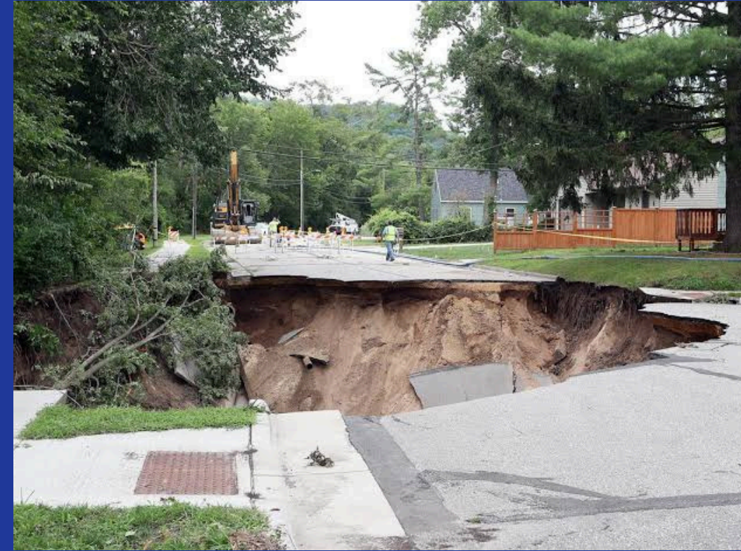
Sinkhole near Myrick Park along Marsh, 2017
