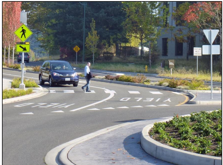
Figure 4: This multilane roundabout provides RRFBs at the pedestrian crossings.
