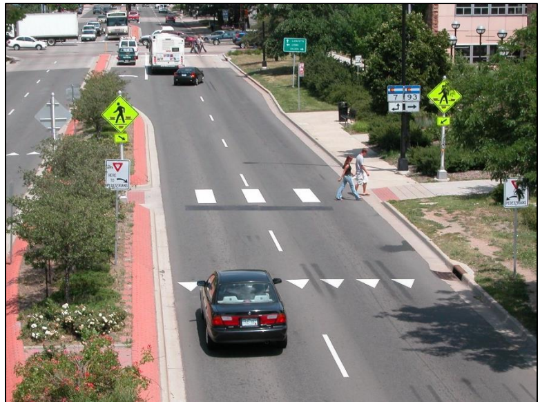
Figure 7: Crossings between roundabouts should include features to improve pedestrian safety and visibility similar to the crossing shown here.
