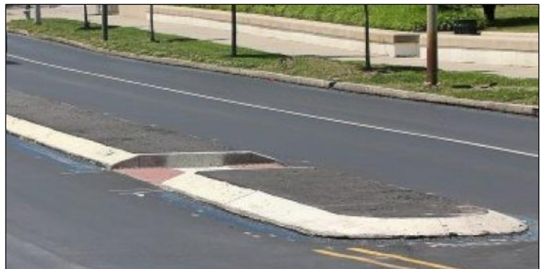
Figure 5: This median uses a mountable curb that allows emergency vehicle access across the median.
