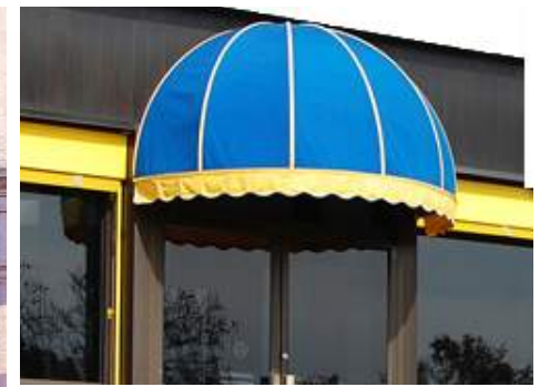
Example of Unacceptable Awning
