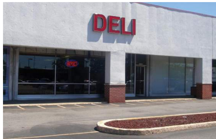
Unacceptable Signage Placement
