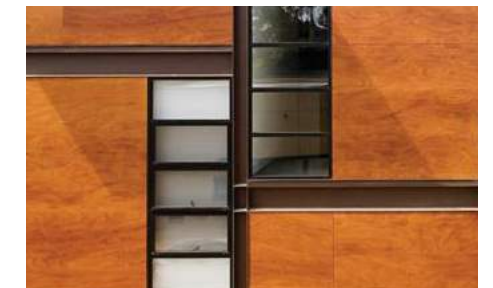
Wood paneling in storefront
