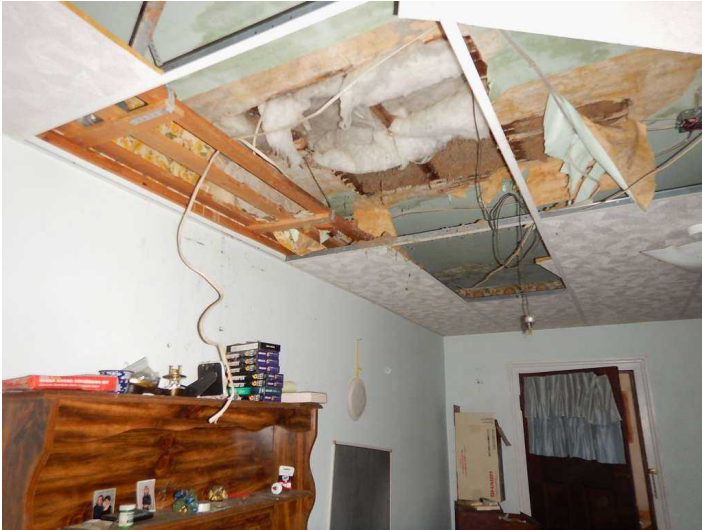
Ceiling Family Room
