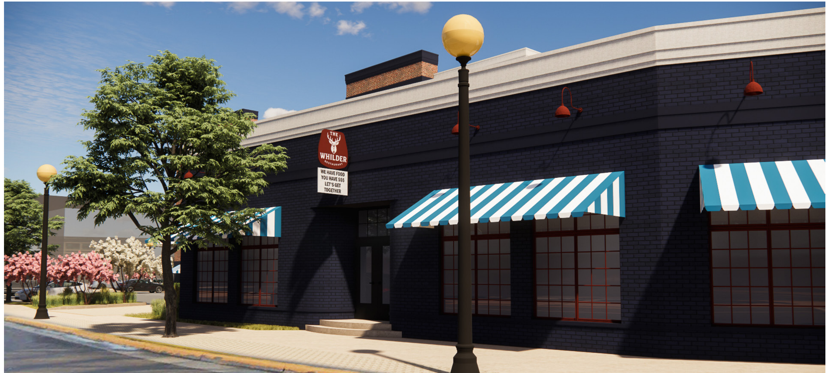
fully painted | updated entry doors and unique feature signage | awnings | new accent lighting (placed in existing locations)
