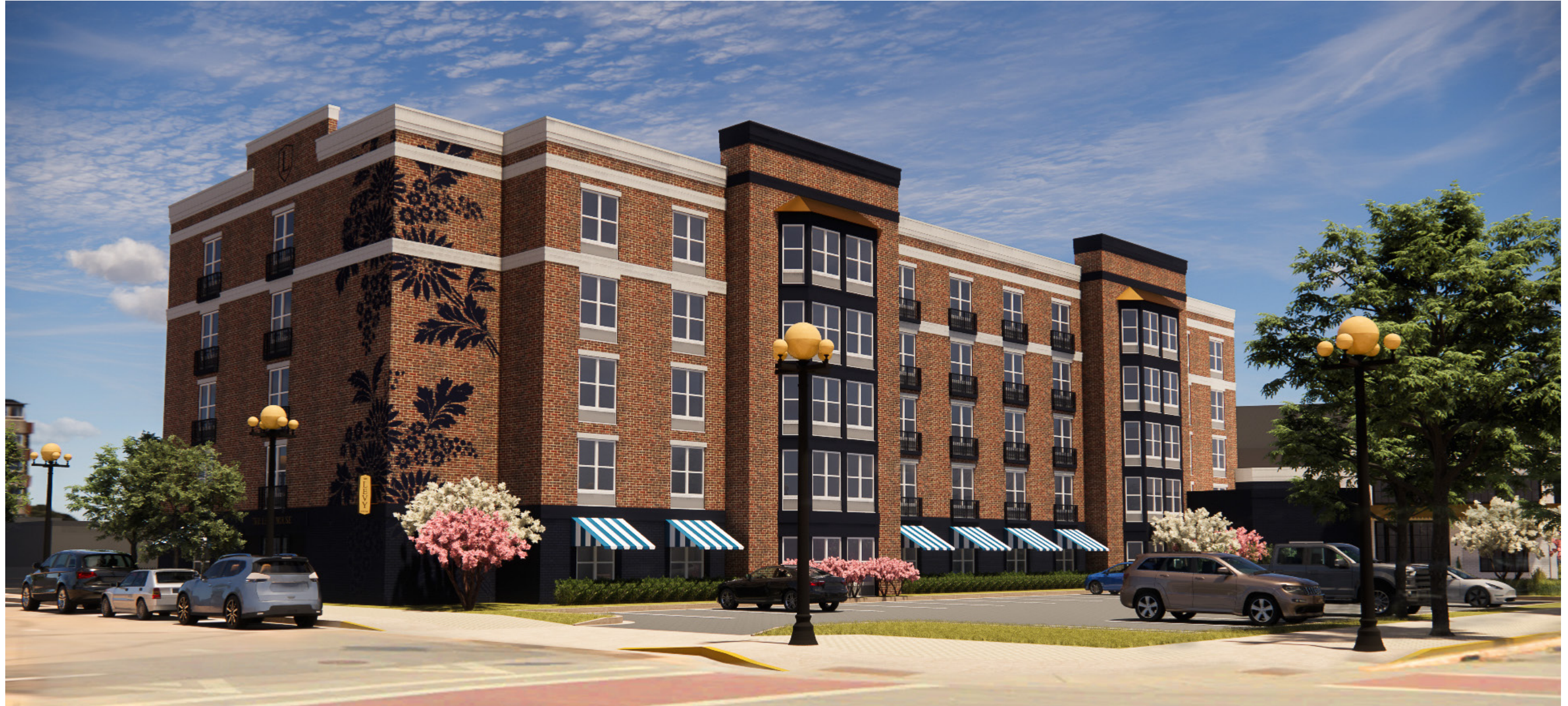
natural brick | faux balconies | updated entry doors and signage | large-scale mural | awnings at street level | dark painted brick at street level | removal of existing peaks
