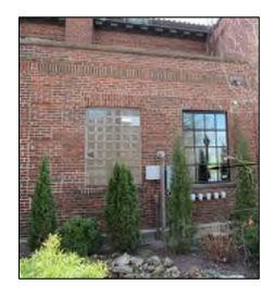
As picture to the right, two of the three existing windows in the lower portion of the west wing will be replaced. The remaining window will be removed and a new door opening will be installed in its place. The existing door an metal stairway will be removed and the opening will be infilled with brick.
