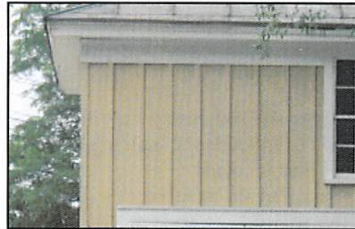
Board & Batten Siding
