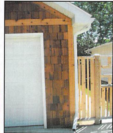
Wood Shingle Siding
