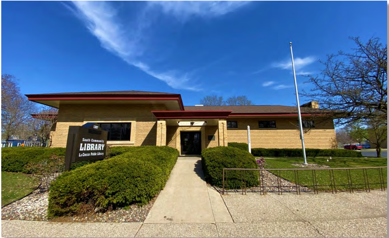
South Branch Library, West Elevation, 2024. Source: David Riel.
