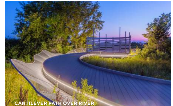
CANTILEVER PATH OVER RIVER
