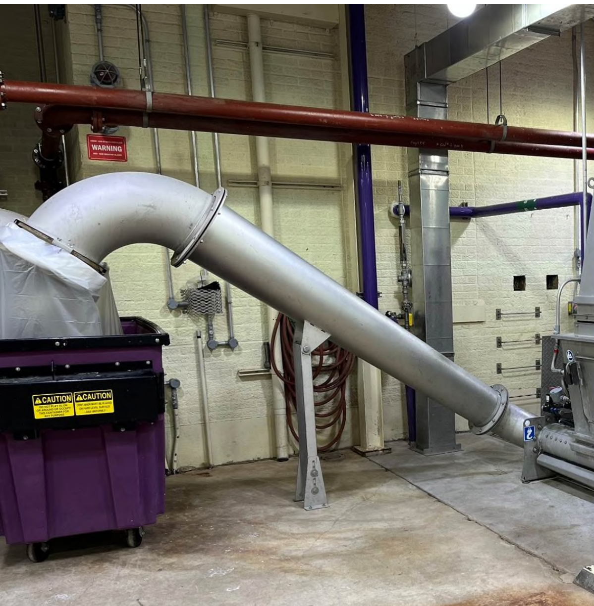
Second influent fine screen and additional compactor.
