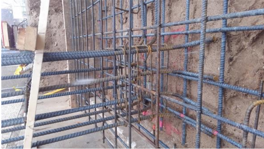
Footing steel reinforcement at gridline 14/E
