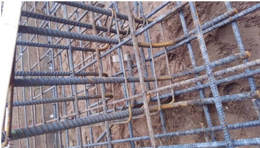
Footings steel reinforcement at gridline 15/E
