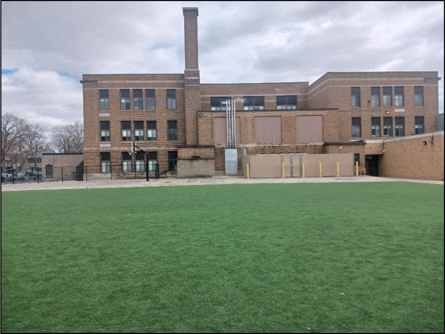
Rear view from 8 th Street showing the final 1-story brick addition.
