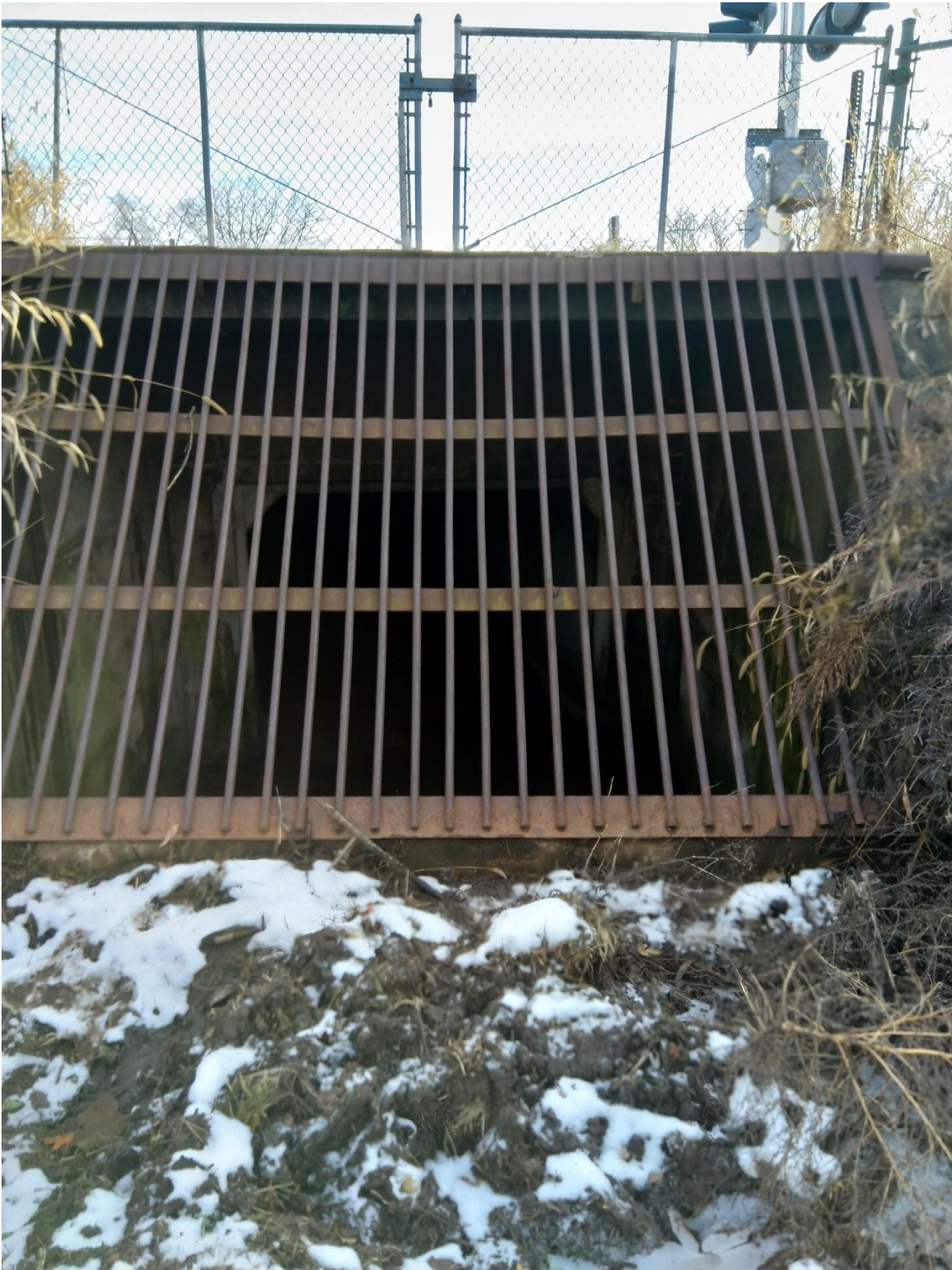
Photo 1 – Grate at entrance to 8x10 foot box culvert under Farnam Street
