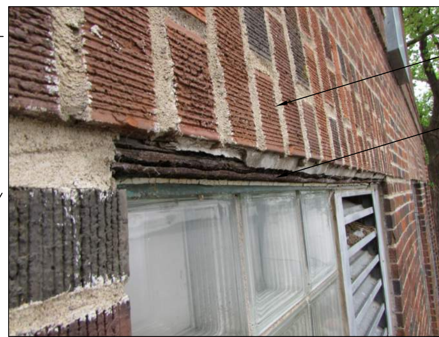
P10 RUSTED LINTEL NO SCALE
