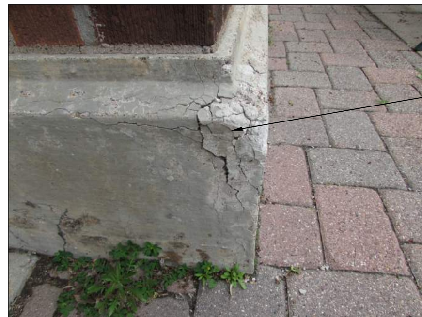
P3 DAMAGED CONCRETE NO SCALE
