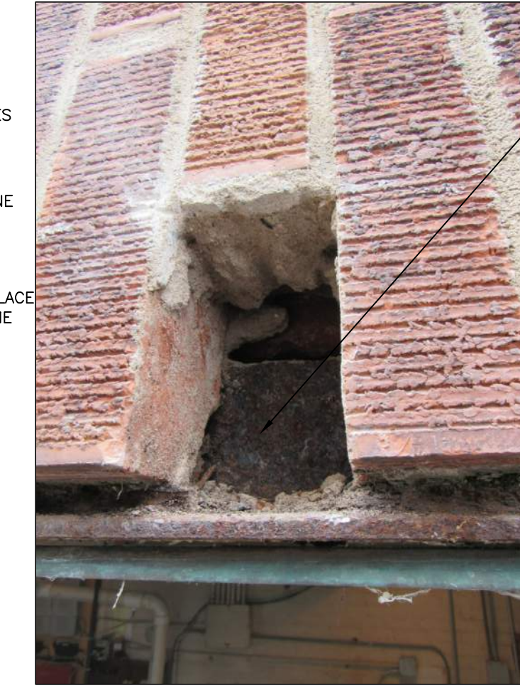
P16 LINTEL DETAIL NO SCALE
