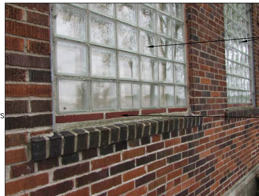
P11 TYP. WINDOW SILL NO SCALE
