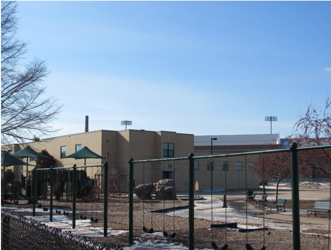
Figure 22 – View of the northeast façade of Emerson School. February 2026.
