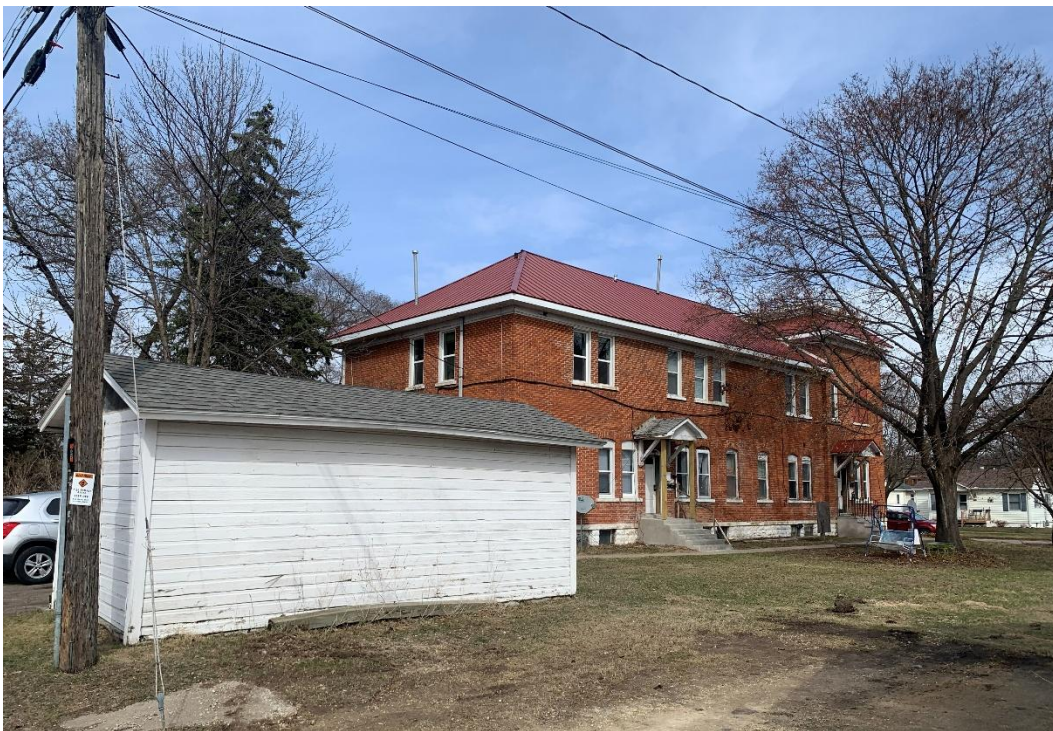
Figure 17 – View of the south and west elevations and garage. March 2026.
