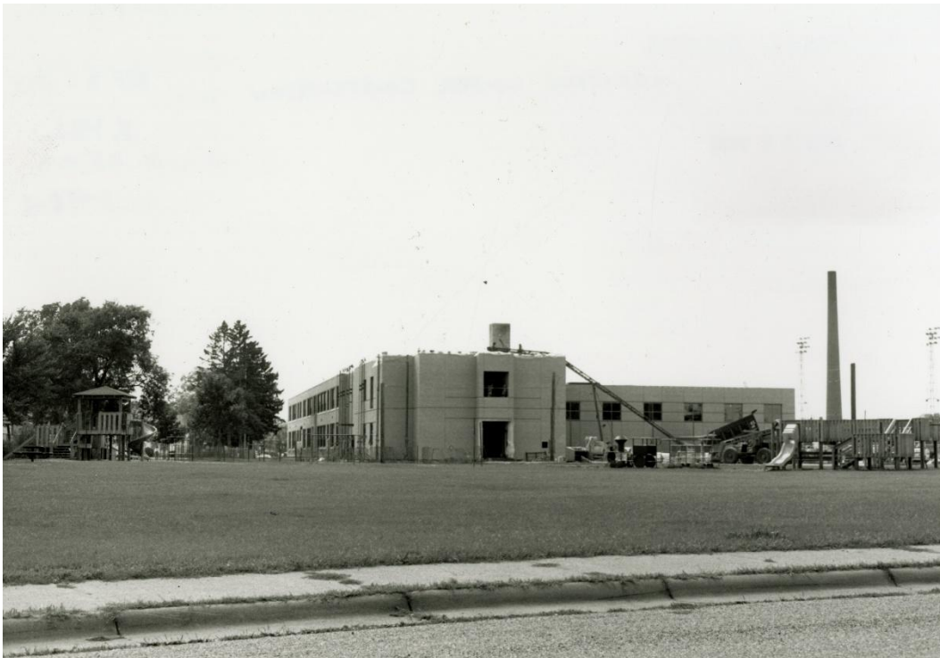
Figure 9 – New north addition at Emerson Orthopedic School looking west. Ca. 1992. Courtesy of University of Wisconsin – La Crosse Murphy Library Special Collections.
