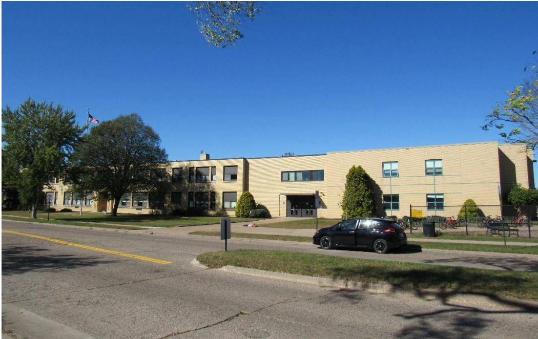
Figure 16 – View of southeast (front) façade of Emerson School. October 2025.
