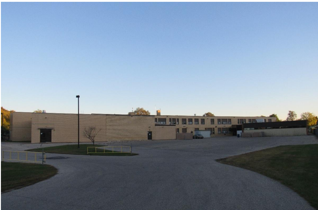
Figure 21 – View of the northwest (back) façade at Emerson School. Looking south at the gym and classroom additions. October 2025.
