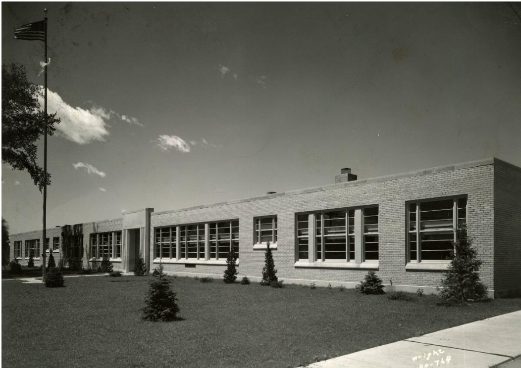
Figure 4 – View looking west from Campbell Street. Ca. 1940. Courtesy of University of Wisconsin – La Crosse Murphy Library Special Collections.
