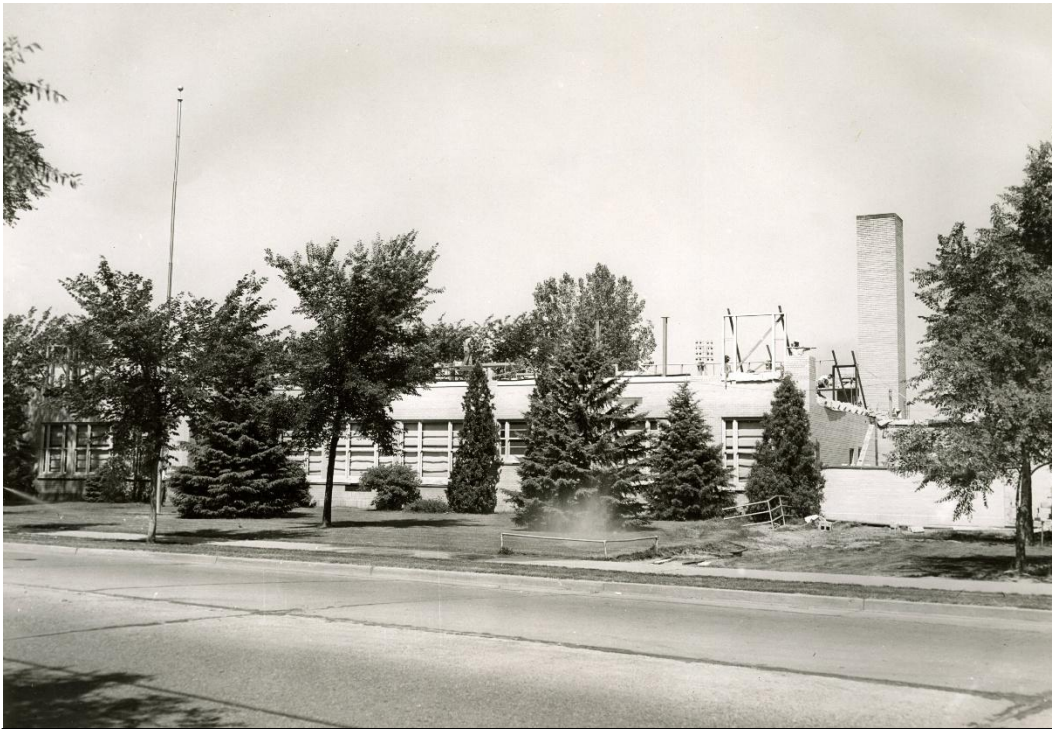
Figure 6 – Second floor construction at Emerson Orthopedic School. Ca. 1956. Courtesy of University of Wisconsin – La Crosse Murphy Library Special Collections.
