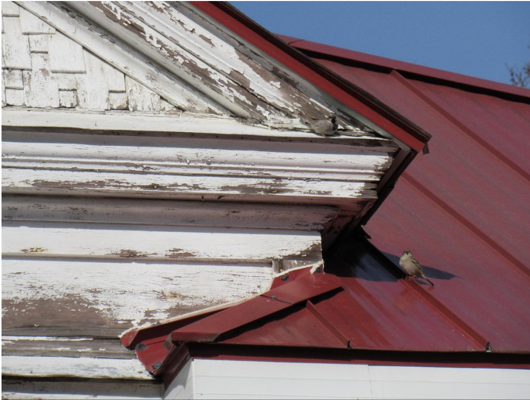
Figure 14 – Eave detail at gable, trim appears to be original. March 2026.
