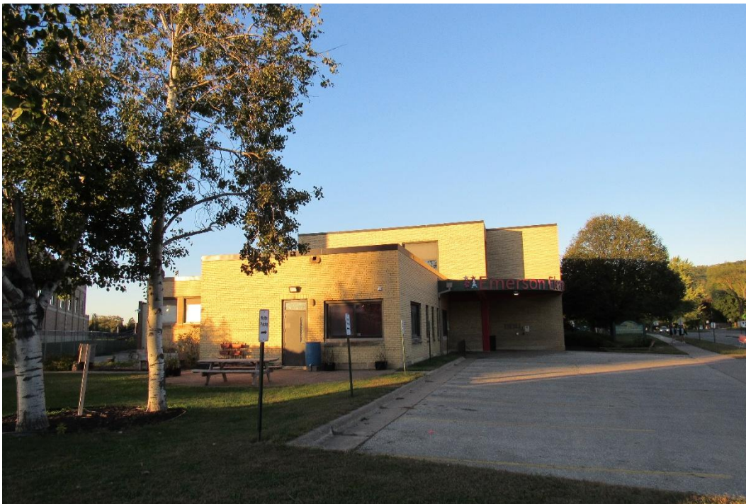
Figure 19 – Main entry and southwest façade looking northeast at Emerson School. October 2025.
