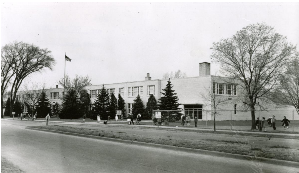
Figure 7 – Second floor completed at Emerson Orthopedic School. Ca. 1956. Courtesy of University of Wisconsin – La Crosse Murphy Library Special Collections.
