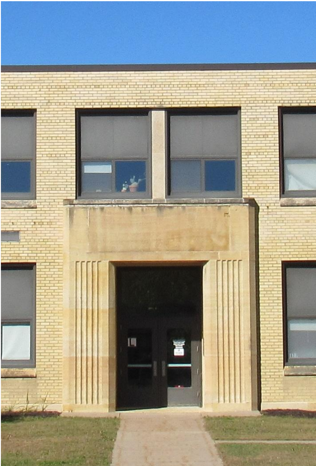
Figure 23 – View of the original main entry at Emerson School. October 2025.
