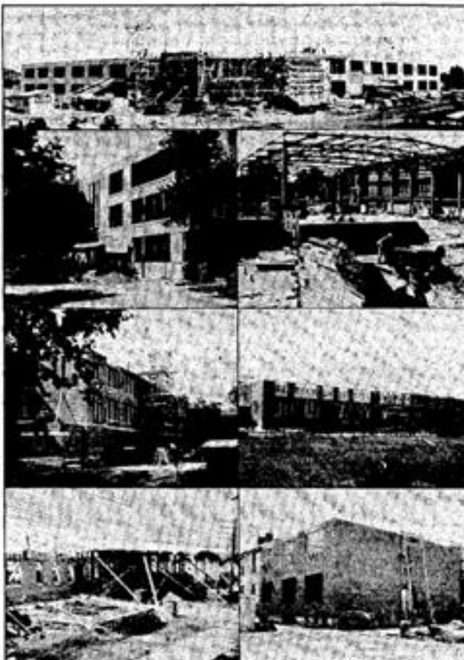
All eight of the new La Crosse school buildings are shown in the above pictures. At the top is the Longfellow Junior high school. The second shows the Vocational school addition, left, and the Logan high school gymnasium-auditorium addition. The third row shows the Aquinas high school addition, left, and the Teachers' college training school. The fourth row shows the Hillview kindergarten-elementary school, left, and the Roosevelt school addition. At the right is the Holy Trinity school addition.
