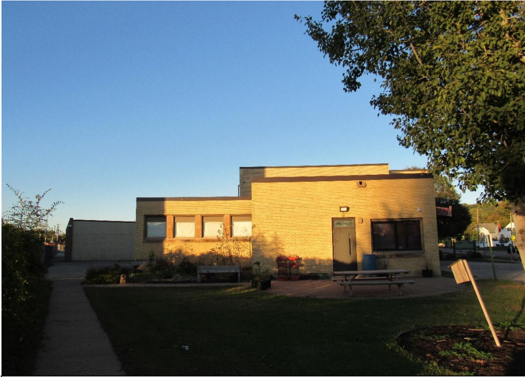
Figure 20 – View of the southwest façade at Emerson School. October 2025.
