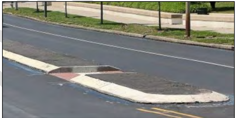
Figure 3: This median uses a mountable curb that allows emergency vehicle access across the median.
