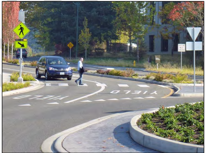
Figure 2: This multilane roundabout provides RRFBs at the pedestrian crossings.
