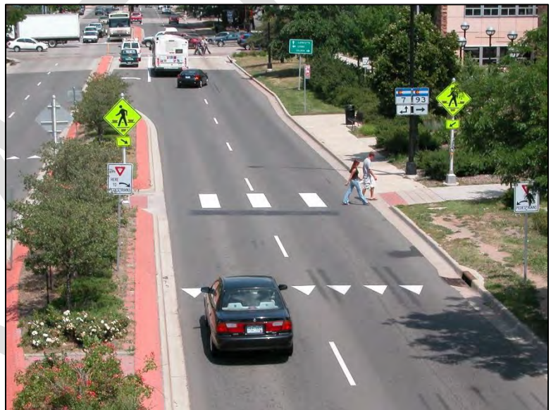
Figure 5: Crossings between roundabouts should include features to improve pedestrian safety and visibility similar to the crossing shown here.
