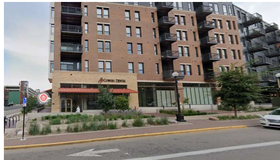
A recent residential building uses more clean, modern materials that are compatible with traditional buildings.
