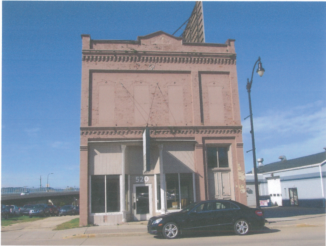
520 Third St. S., east (front) façade, facing west.
