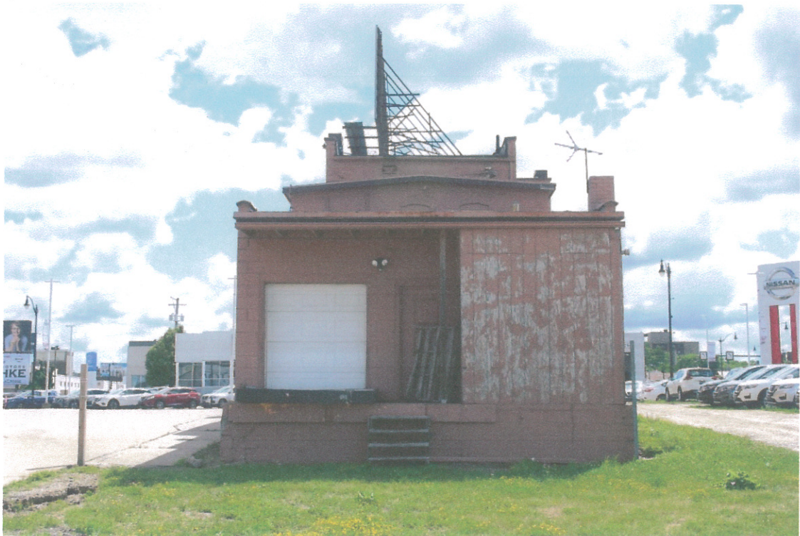
520 Third St. S., west/back façade, facing east.
