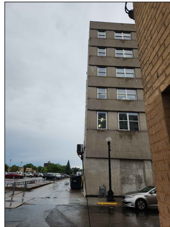
PROPOSED AIR INTAKE WILL BE HIDDEN BY EXISTING A/C UNITS FROM VIEW FROM JAY ST
