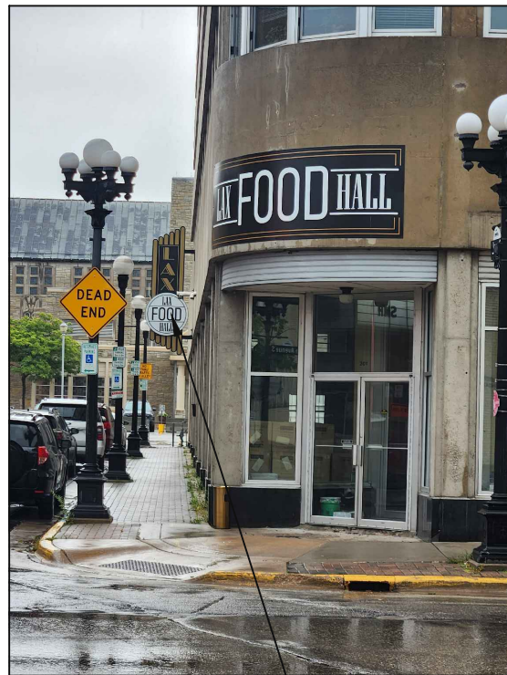
PROPOSED HOOD DUCT EXHAUST FANS WILL BE HIDDEN BY EXISTING SIGN FROM VIEW FROM 5TH AVE
