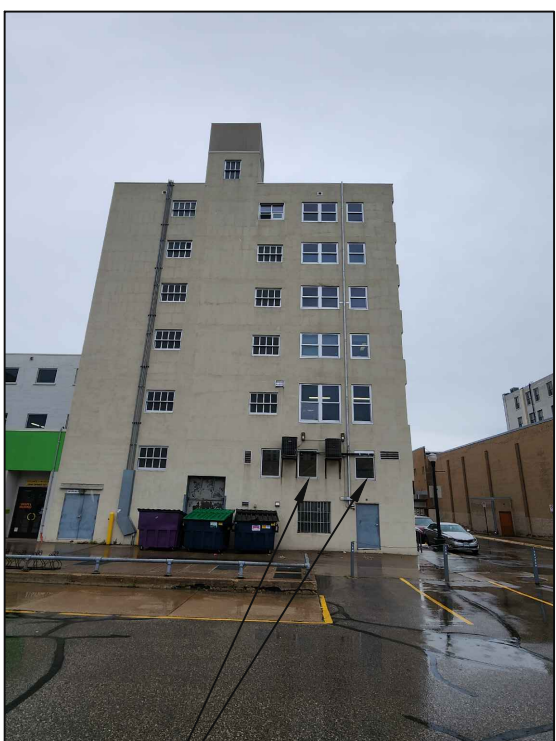
THESE TWO WINDOWS WILL BE USED AS AIR INTAKE
